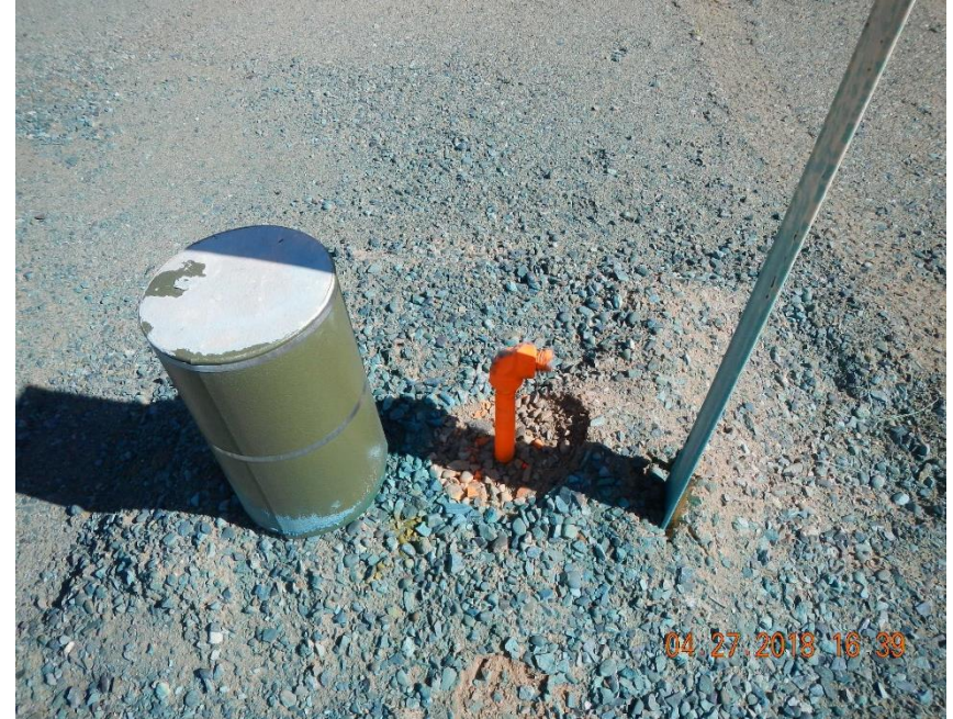
1" steel riser painted orange with insulated cover.
