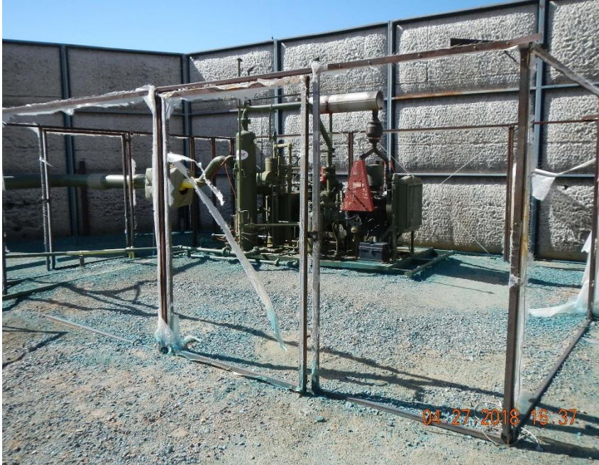
Skid mounted compressor with wind screen frame.
