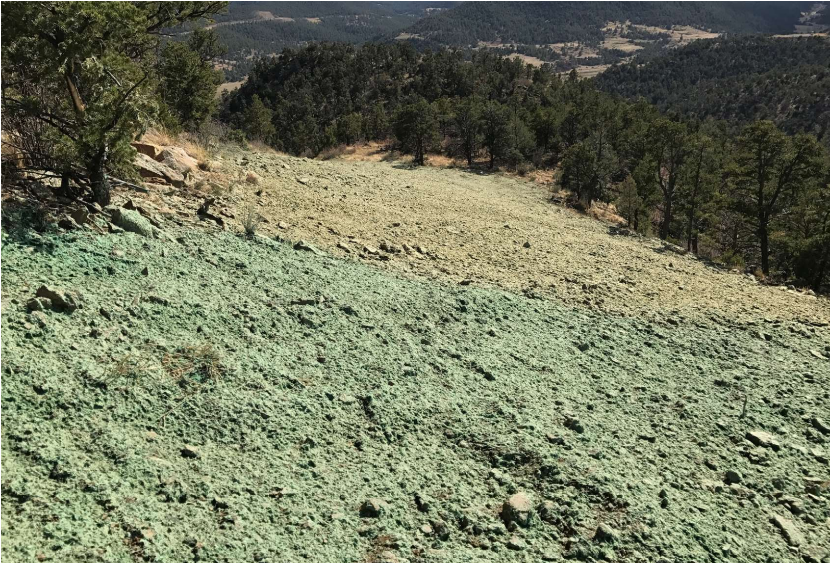
PHOTO 6: FACING SOUTH, THE ACCESS ROAD/PIPELINE R.O.W. WAS RECONTOURED TO MATCH THE SURROUNDING TERRAIN. GRADING TECHNIQUES WERE INSTALLED ON THE CONTOUR TO PROMOTE GROUND INFILTRATION AND PREPARE THE SOIL FOR SEEDING. THE EARTH DISTURBANCE WAS STABILIZED BY HYDRO-SEEDING USING AN APPROVED HILL RANCH SEED MIX TO PROMOTE THE ESTABLISHMENT OF VEGETATION.
