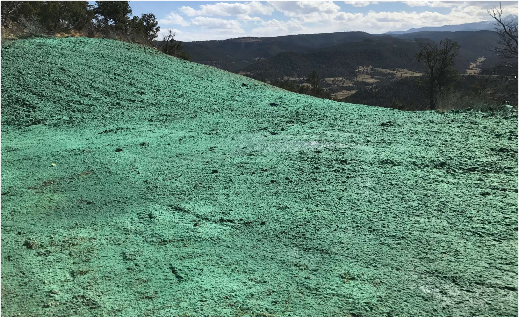
PHOTO 7: NORTHEAST END OF RECLAMATION ADJACENT TO THE MAIN LEASE ROAD IN LOPEZ CANYON. THE ACCESS ROAD/ PIPELINE R.O.W. WAS RECONTOURED TO MATCH THE SURROUNDING TERRAIN. GRADING TECHNIQUES WERE INSTALLED ON THE CONTOUR TO PROMOTE GROUND INFILTRATION AND PREPARE THE SOIL FOR SEEDING. THE EARTH DISTURBANCE WAS STABILIZED BY HYDRO-SEEDING USING AN APPROVED HILL RANCH SEED MIX TO PROMOTE THE ESTABLISHMENT OF VEGETATION.
