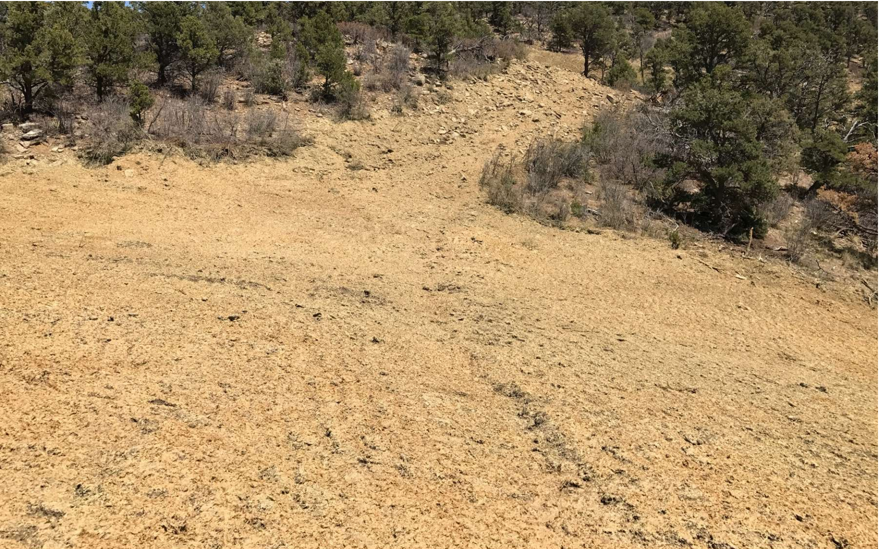
PHOTO 2: VIEW NORTHEAST ALONG THE RECLAIMED WELL PAD AND ACCESS ROAD. THE ACCESS ROAD AND WELL PAD WERE RECONTOURED TO MATCH THE SURROUNDING TERRAIN WHICH CORRECTED THE EROSION ISSUES. GRADING TECHNIQUES WERE INSTALLED ON THE CONTOUR TO PROMOTE GROUND INFILTRATION AND PREPARE THE SOIL FOR SEEDING. THE EARTH DISTURBANCE WAS STABILIZED BY HYDRO-SEEDEDING USING AN APPROVED HILL RANCH SEED MIX TO PROMOTE THE ESTABLISHMENT OF VEGETATION.
