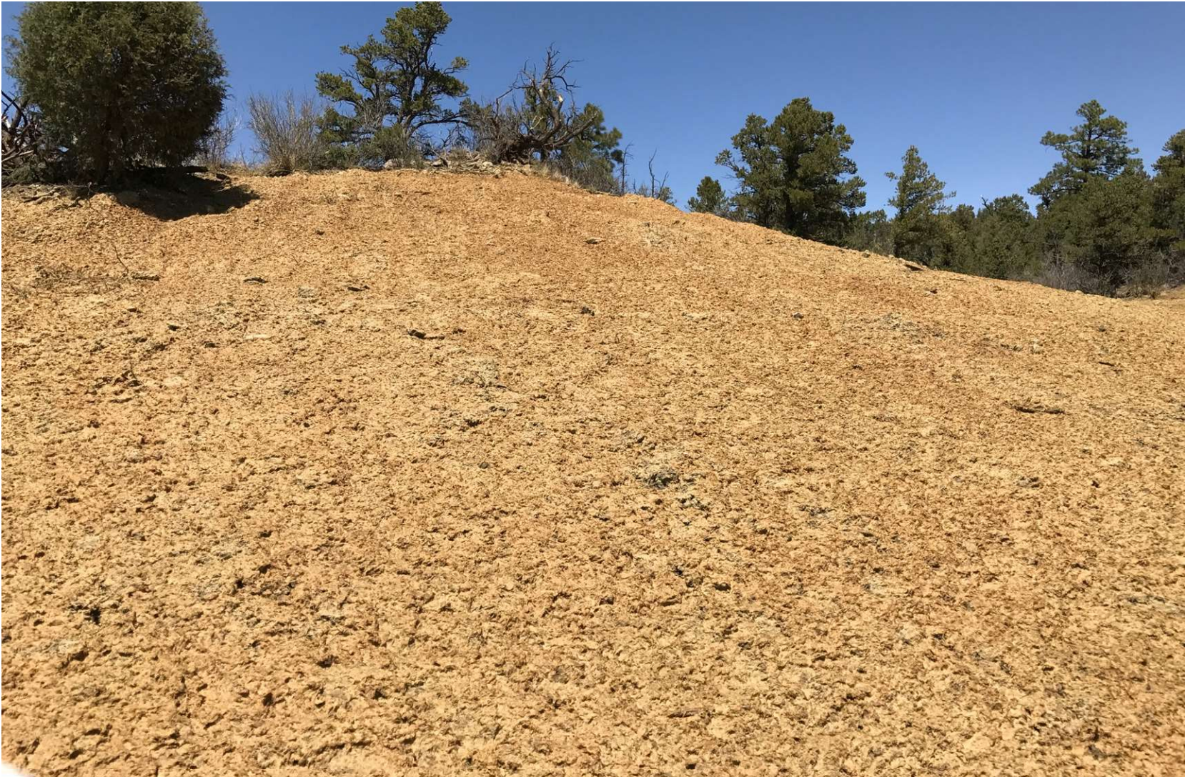
PHOTO 4: FACING NORTHWEST AT THE RECLAIMED CUT SLOPE OF WELL PAD. THE WELL PAD WAS RECONTOURED TO MATCH THE SURROUNDING TERRAIN. GRADING TECHNIQUES WERE INSTALLED ON THE CONTOUR TO PROMOTE GROUND INFILTRATION AND PREPARE THE SOIL FOR SEEDING. THE EARTH DISTURBANCE WAS STABILIZED BY HYDRO-SEEDING USING AN APPROVED HILL RANCH SEED MIX TO PROMOTE THE ESTABLISHMENT OF VEGETATION.
