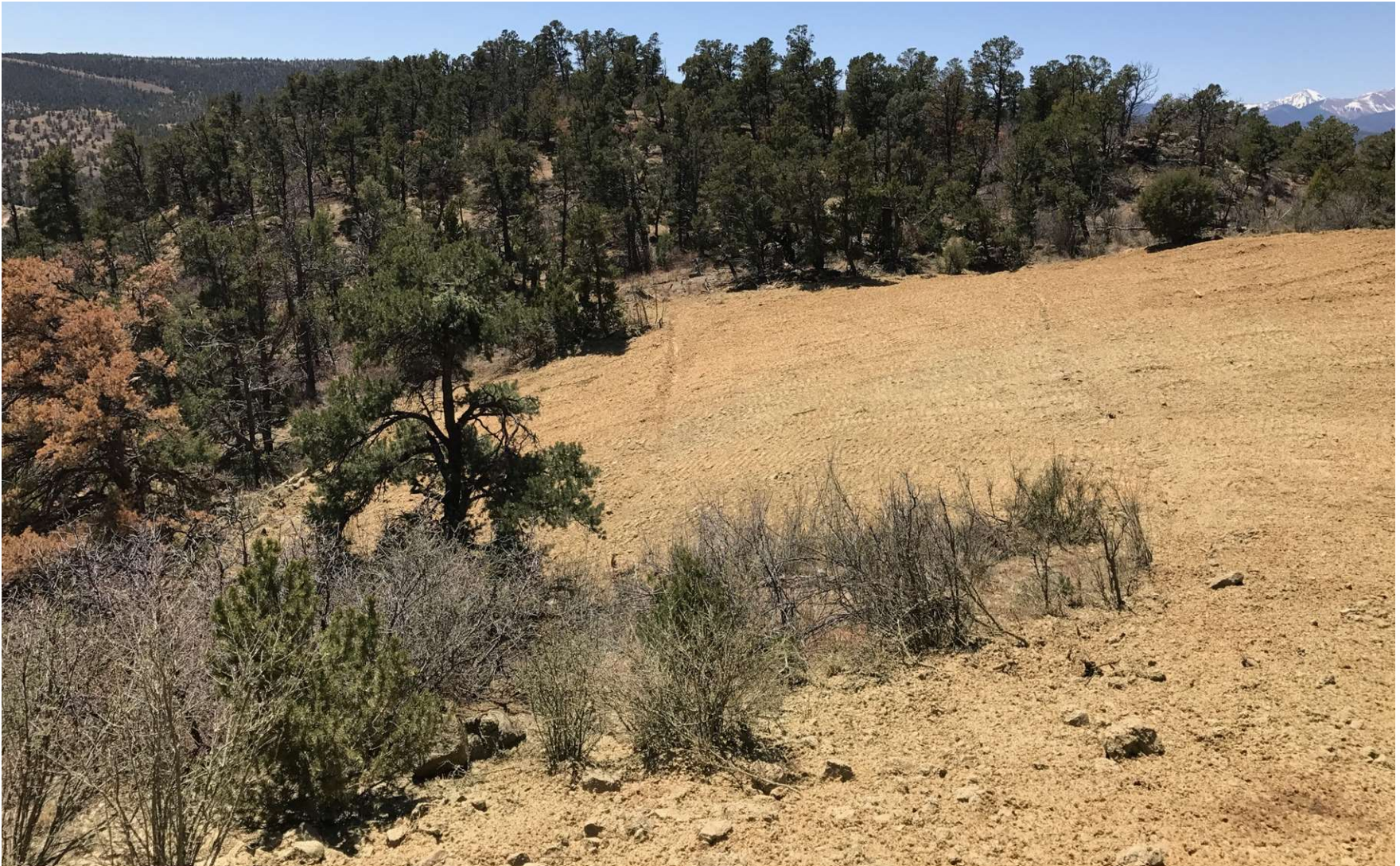
PHOTO 1: OVERVIEW OF LOCATION TO WEST. THE ACCESS ROAD AND WELL PAD WERE RECONTOURED TO MATCH THE SURROUNDING TERRAIN. THIS PROCESS ALLOWED FOR SOIL DECOMPACTION. THE TOPSOIL STOCKPILE WAS USED TO RECLAIM LOCATION. GRADING TECHNIQUES WERE INSTALLED ON THE CONTOUR TO PROMOTE GROUND INFILTRATION AND PREPARE THE SOIL FOR SEEDING. THE EARTH DISTURBANCE WAS STABILIZED BY HYDRO-SEEDING USING AN APPROVED HILL RANCH SEED MIX TO PROMOTE THE ESTABLISHMENT OF VEGETATION. ALL PIPING AND DEBRIS WERE REMOVED FROM LOCATION.
