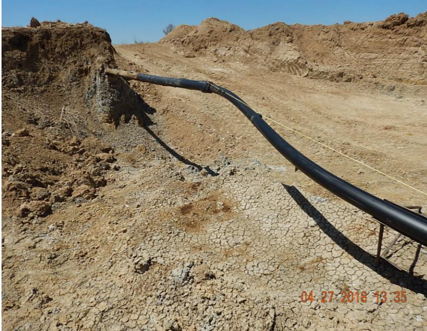
View of flowline repair in progress; area where poly has been stung (slip lined) in to existing pipe (w tracer wire)
