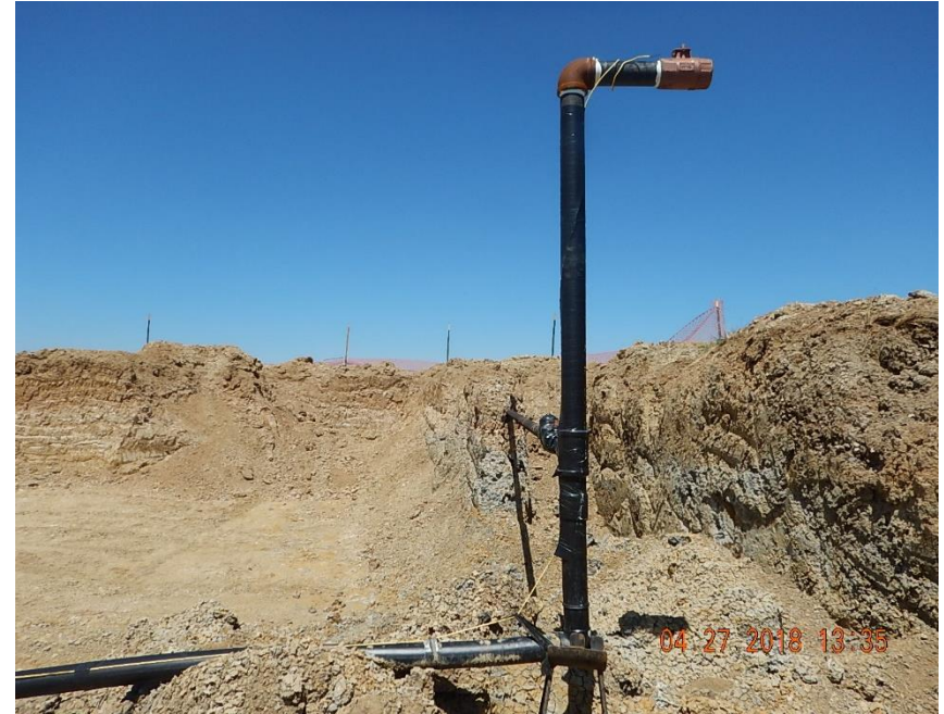
View of flowline repair; in area of well tie in and installation of riser/ valve set
