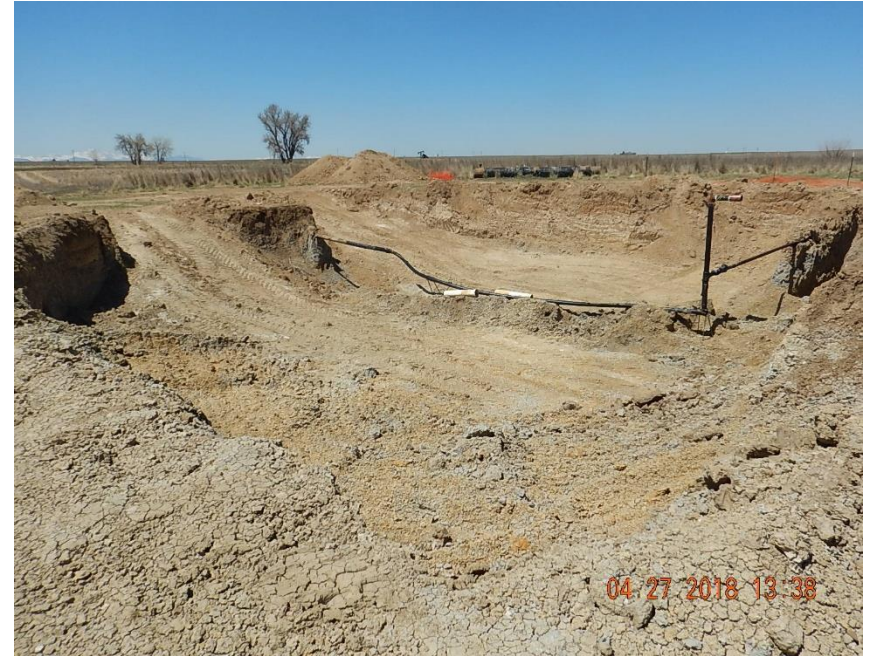
View of excavation and flowline repair work in progress Looking North
