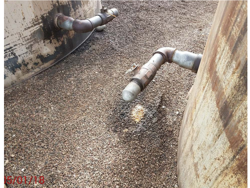
Location photo # 4, Stained material in tank battery, leaking valve
