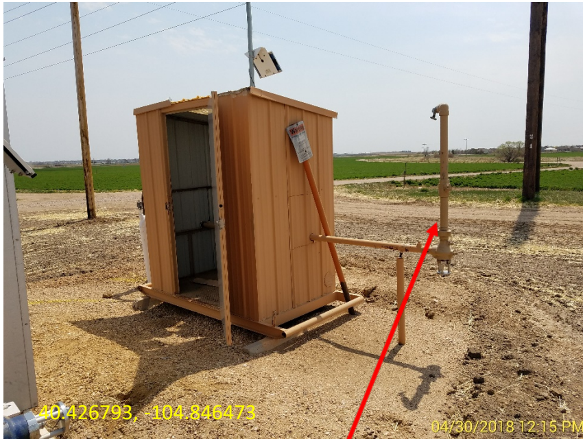
Unused gas meter run Photo #2 Facing SE Line is disconnected
