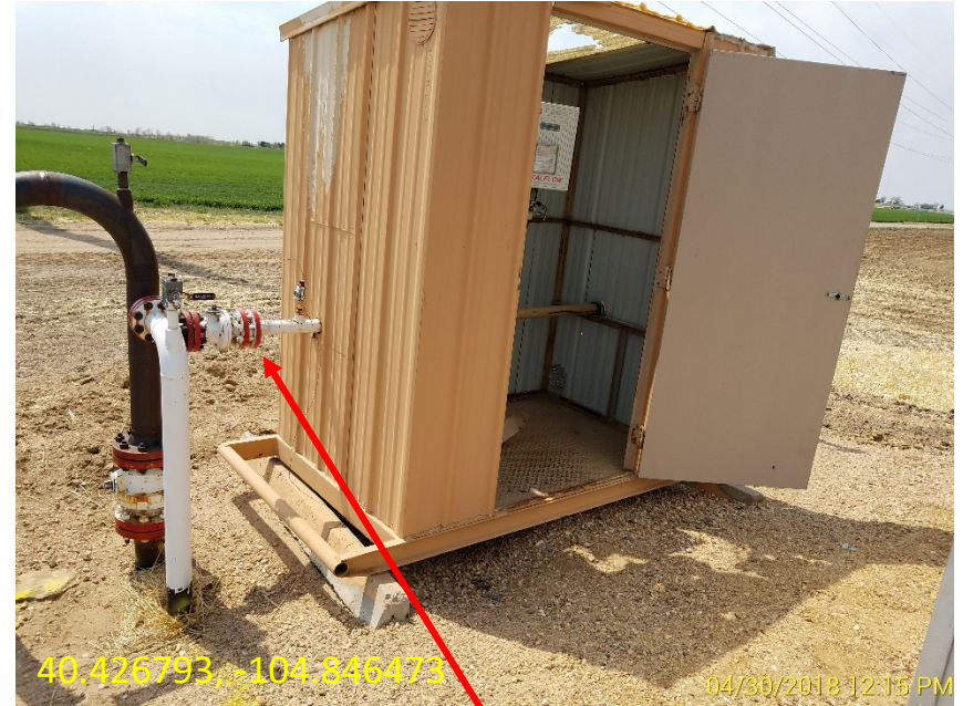
Unused gas meter run Photo #1 Facing SW Valve is shut
