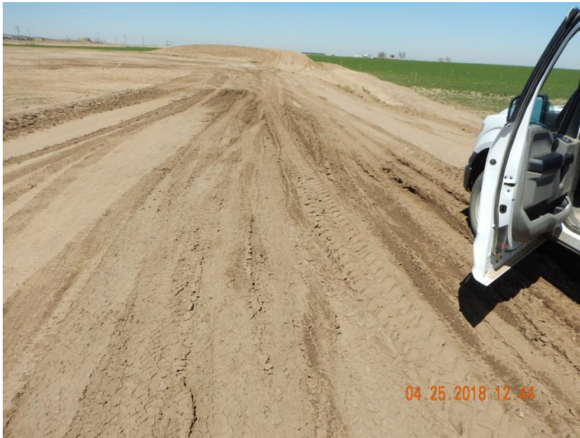
Photo 1. Photo taken from the entrance of the location, facing North. Operator has failed to install a vehicle tracking device to prevent track of material offsite.
