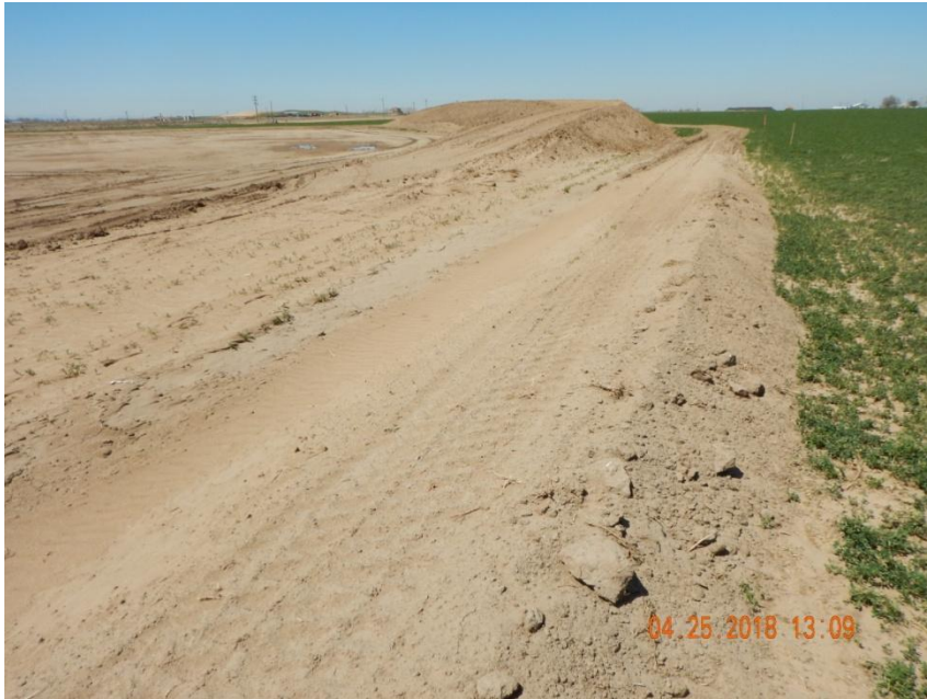
Photo 3. Photo taken from the eastern perimeter of the location, facing North. Ditch and berm BMP has been installed along the entire perimeter of the location. Portions of the berm do not appear to be stabilized. An unconsolidated berm BMP is not a proper functioning BMP. Photo also illustrates ditch BMP filling up with fines from unconsolidated soil material from the well pad. Appears topsoil is being stored along the northeastern and southwestern perimeter of the location.
