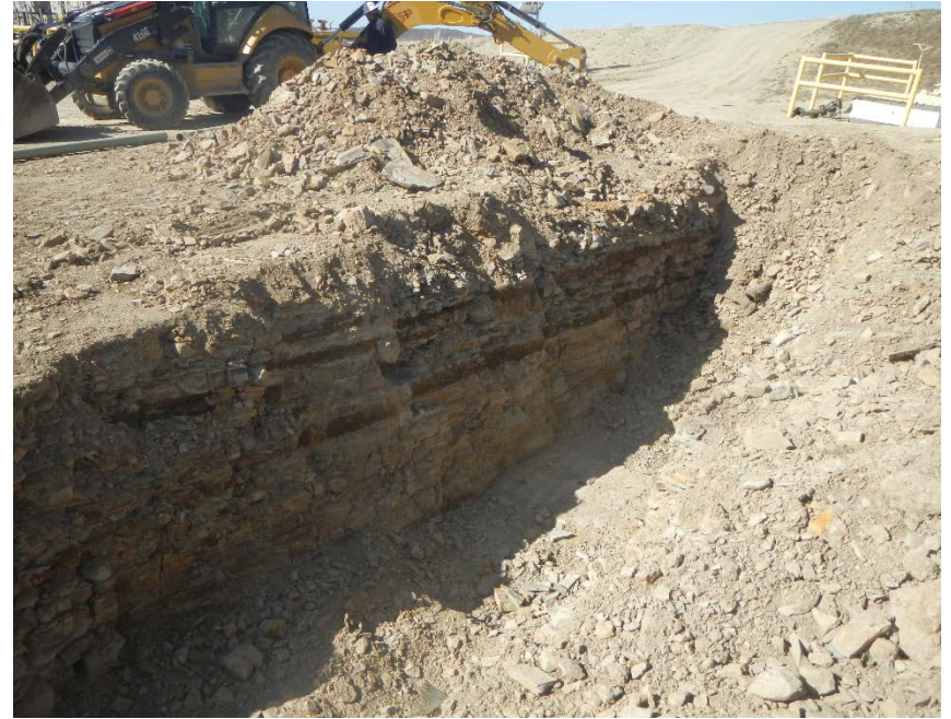
PipeTrench bed looking West, Pipe bedded in friable sandstone/shale.
