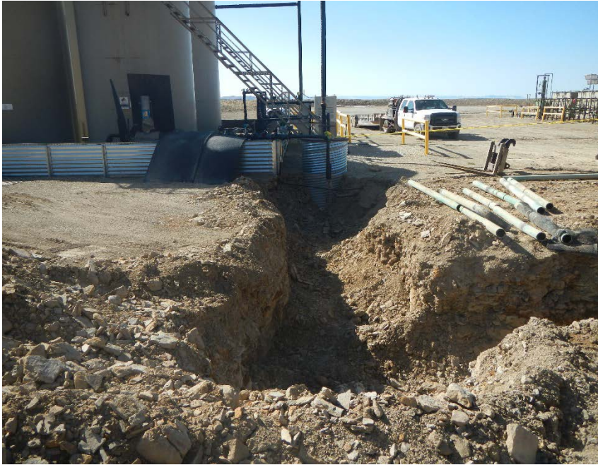
NE corner of pipeline looking South, Compromised 4" line has been removed
