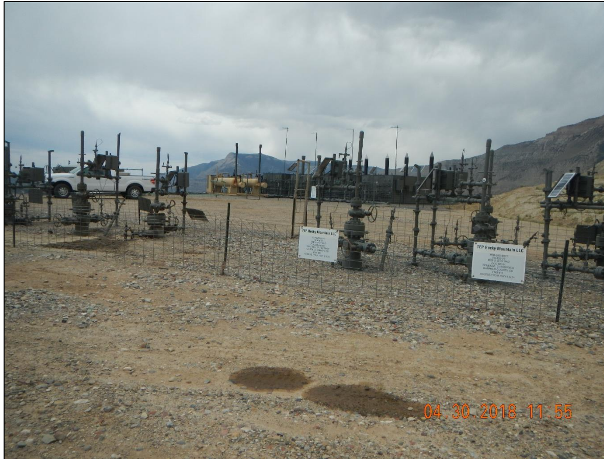
Stained ground in front well head fencing.
