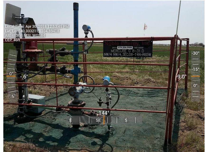
Wellhead after corrective action completed
