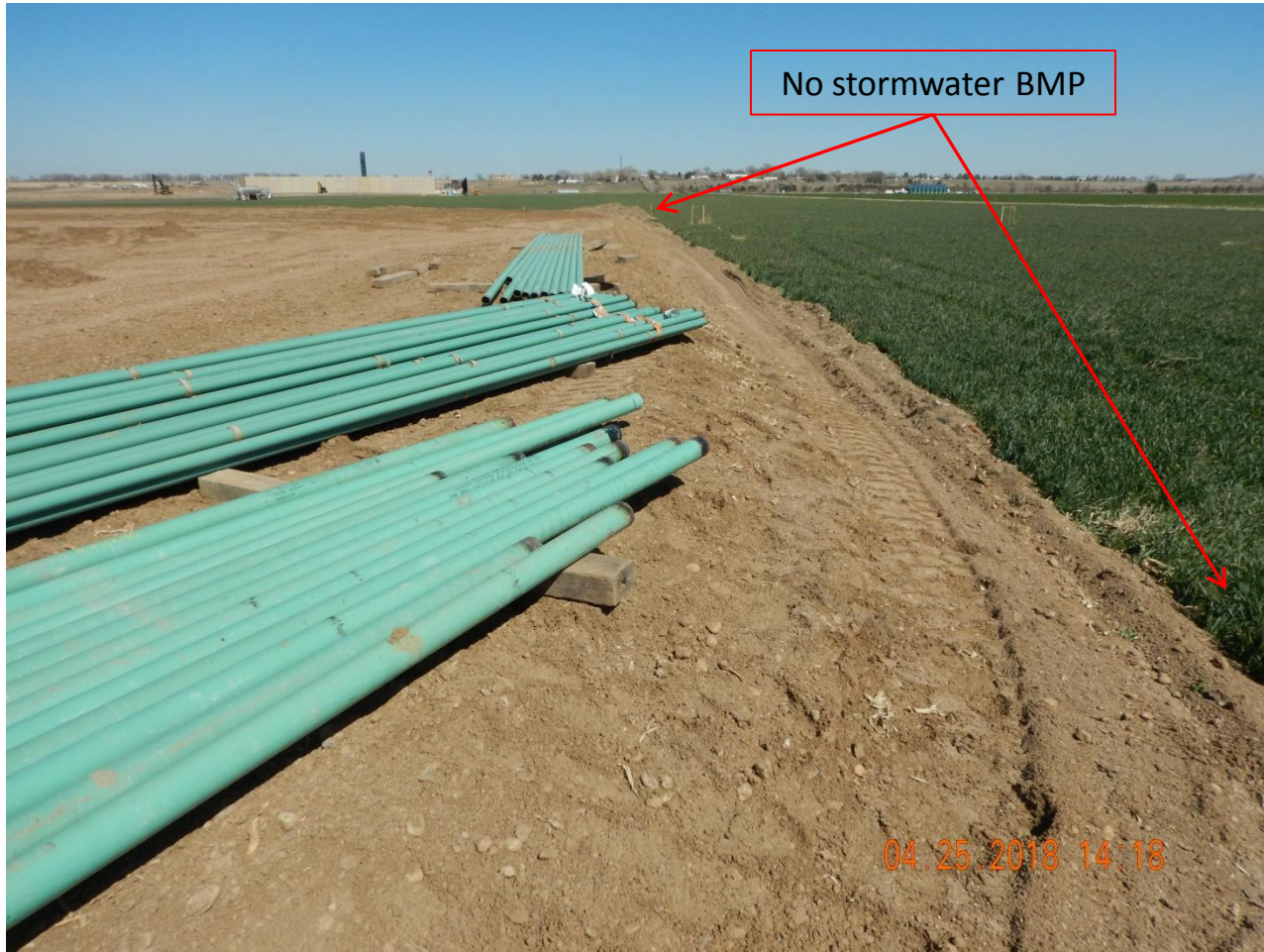
Photo 1. Photo taken from the southwest perimeter of the location, facing East. Operator failed to install stormwater BMPs during construction operations.
