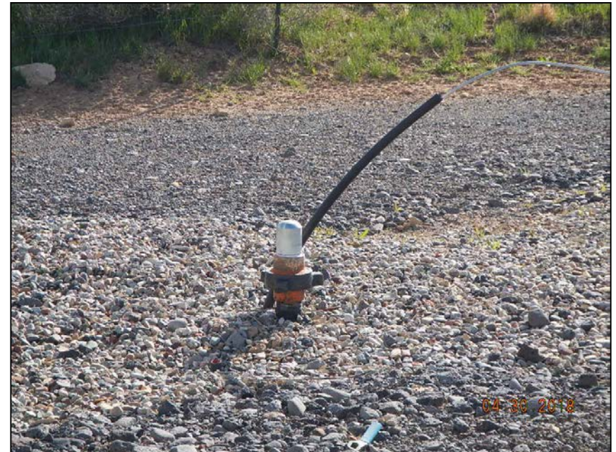
Photo 2. Flowline painted and closed with bull plug..
