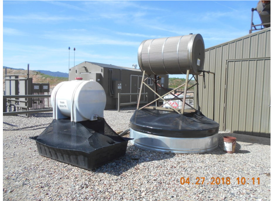
Injection pump housings. Chemical with secondary containment.
