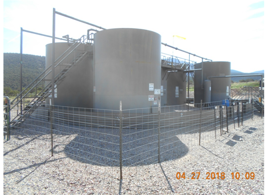
SE production tank battery
