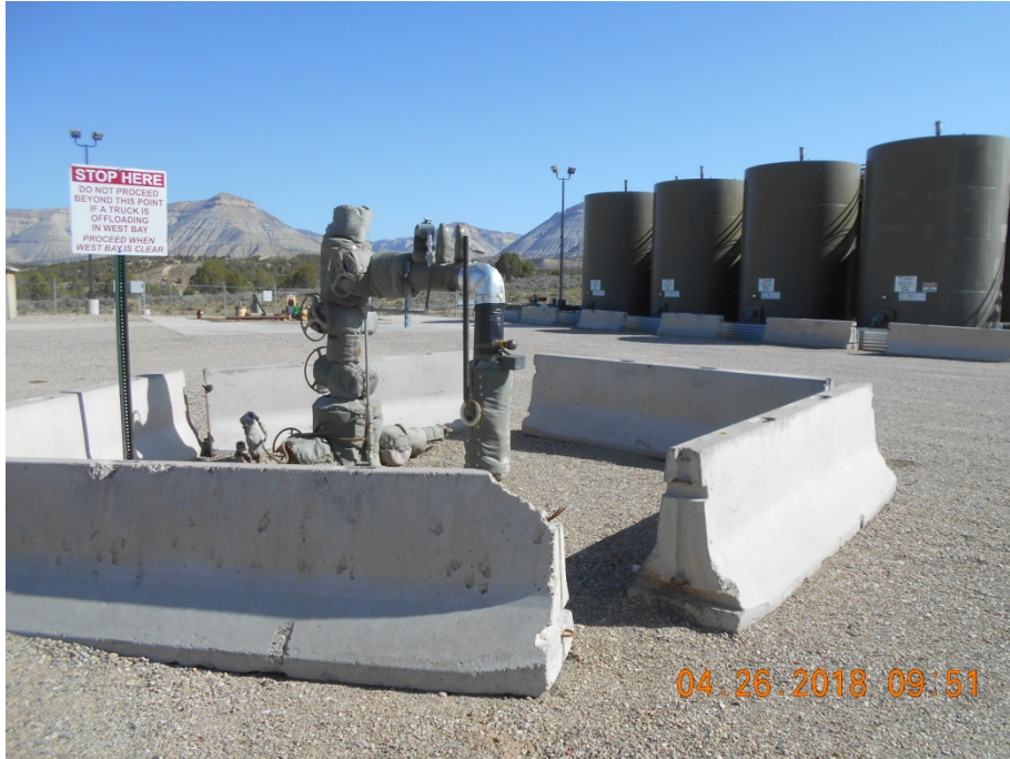
Wellheads with fencing
