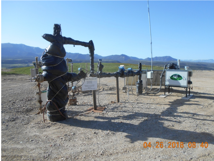
Wellhead with line heater.
