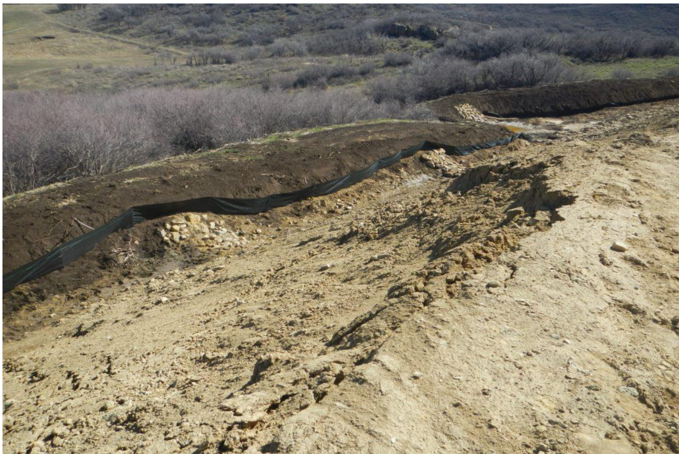
Photo#3: View of Sloughed area of fill slope from top of Pad to base of slope.
