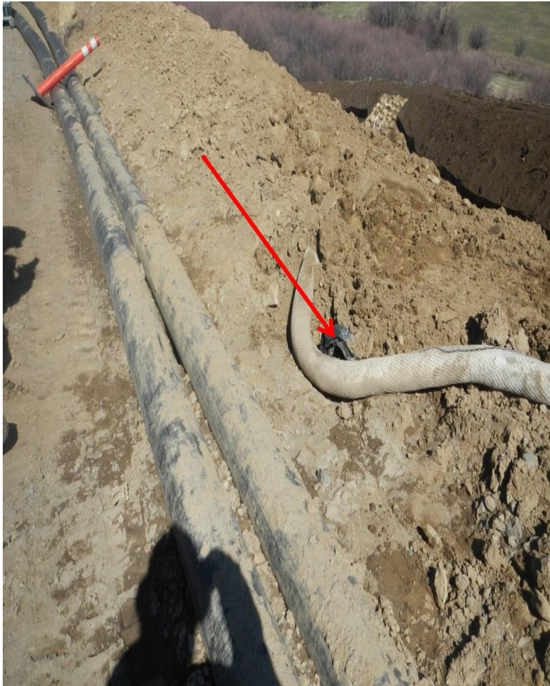
Photo#6: Drain on Southeast edge area of pad. Arrow indicates flexible pipe outlet position.
