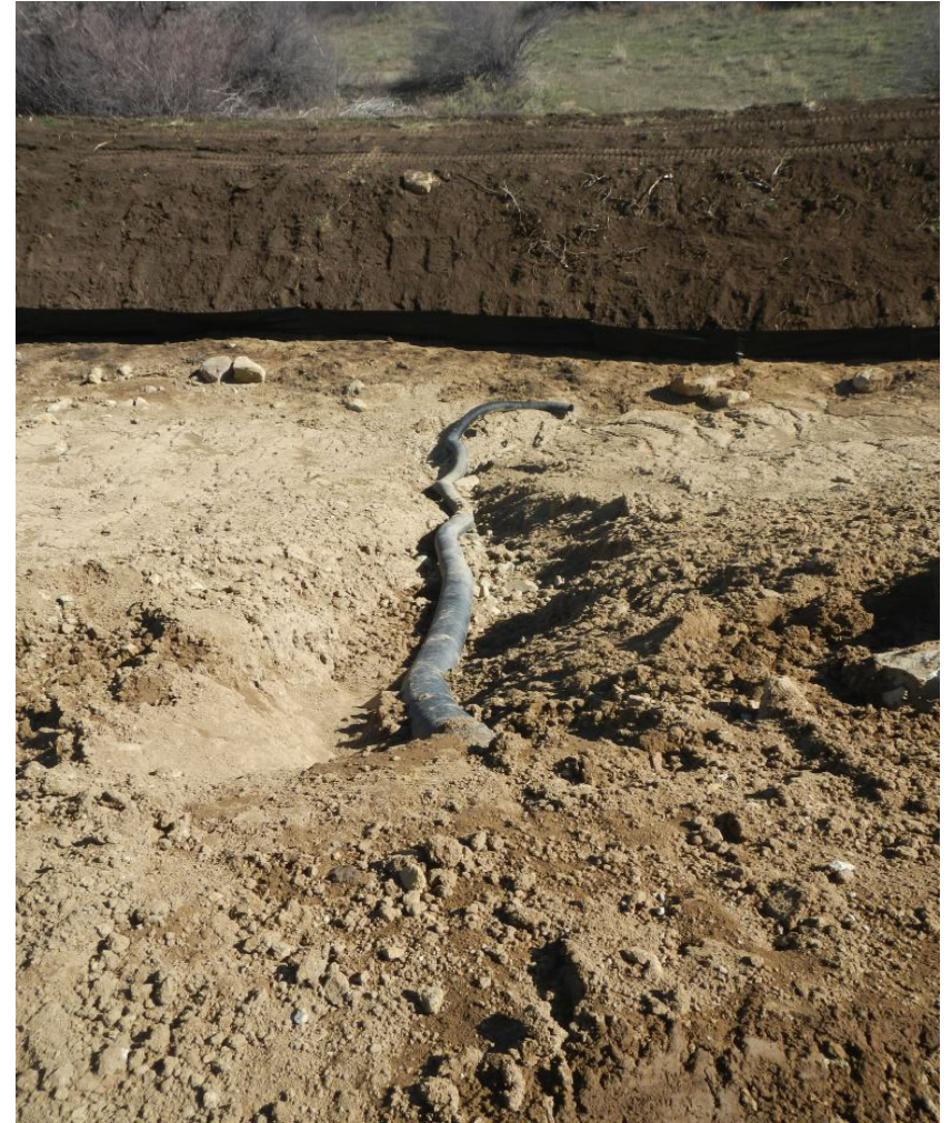
Photo#7 Flexible pipe draining to base of fill slope from Photo#6
