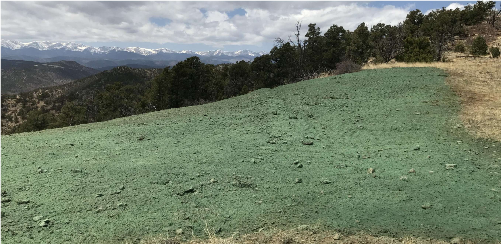
PHOTO 1 : GOLDEN EAGLE MINE NW-3-6-95 RECLAMATION FACING NORTH. THE WELL PAD WAS RECONTOURED TO MATCH THE SURROUNDING TERRAIN. GRADING TECHNIQUES WERE INSTALLED ON THE CONTOUR TO PROMOTE GROUND INFILTRATION AND PREPARE THE SOIL FOR SEEDING. THE EARTH DISTURBANCE WAS STABILIZED BY HYDRO-SEEDING USING AN APPROVED HILL RANCH SEED MIX TO PROMOTE THE ESTABLISHMENT OF VEGETATION. THE TOP SOIL STOCKPILE WAS UTILIZED DURING RECLAMATION ACTIVITIES. (2) WATER BARS WERE INSTALL TO REDUCE RUN OFF VELOCITY. A DIRT BERM WAS INSTALLED DOWN GRADIENT OF THE PROJECT TO PROVIDE PERIMETER SEDIMENT CONTROL.
