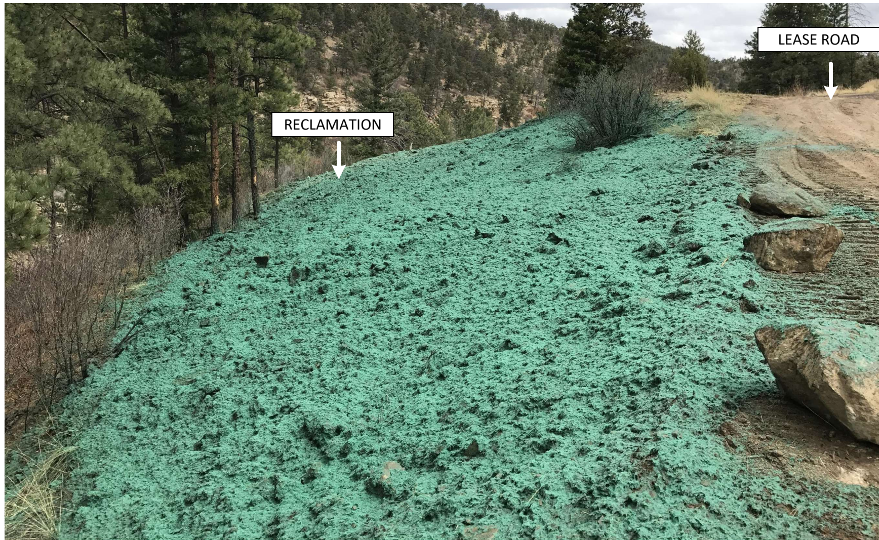
PHOTO 13 : INTERSECTION OF THE ACCESS ROAD RECLAMATION AND THE LEASE ROAD GOING TO THE PRODUCING WELL GOLDEN EAGLE 20-09 API # 071-08803. THE LOWER ROAD WAS RECONTOURED TO MATCH THE SURROUNDING TERRAIN. SOIL ROUGHENING WAS USED TO PROMOTE GROUND INFILTRATION AND PREPARE THE SOIL FOR SEEDING. THE EARTH DISTURBANCE WAS STABILIZED BY HYDRO-SEEDING USING AN APPROVED HILL RANCH SEED MIX TO PROMOTE THE ESTABLISHMENT OF VEGETATION. ARMOR WAS PLACED AT THE END OF THE RECLAMATION TO DETER VEHICLE ACCESS.
