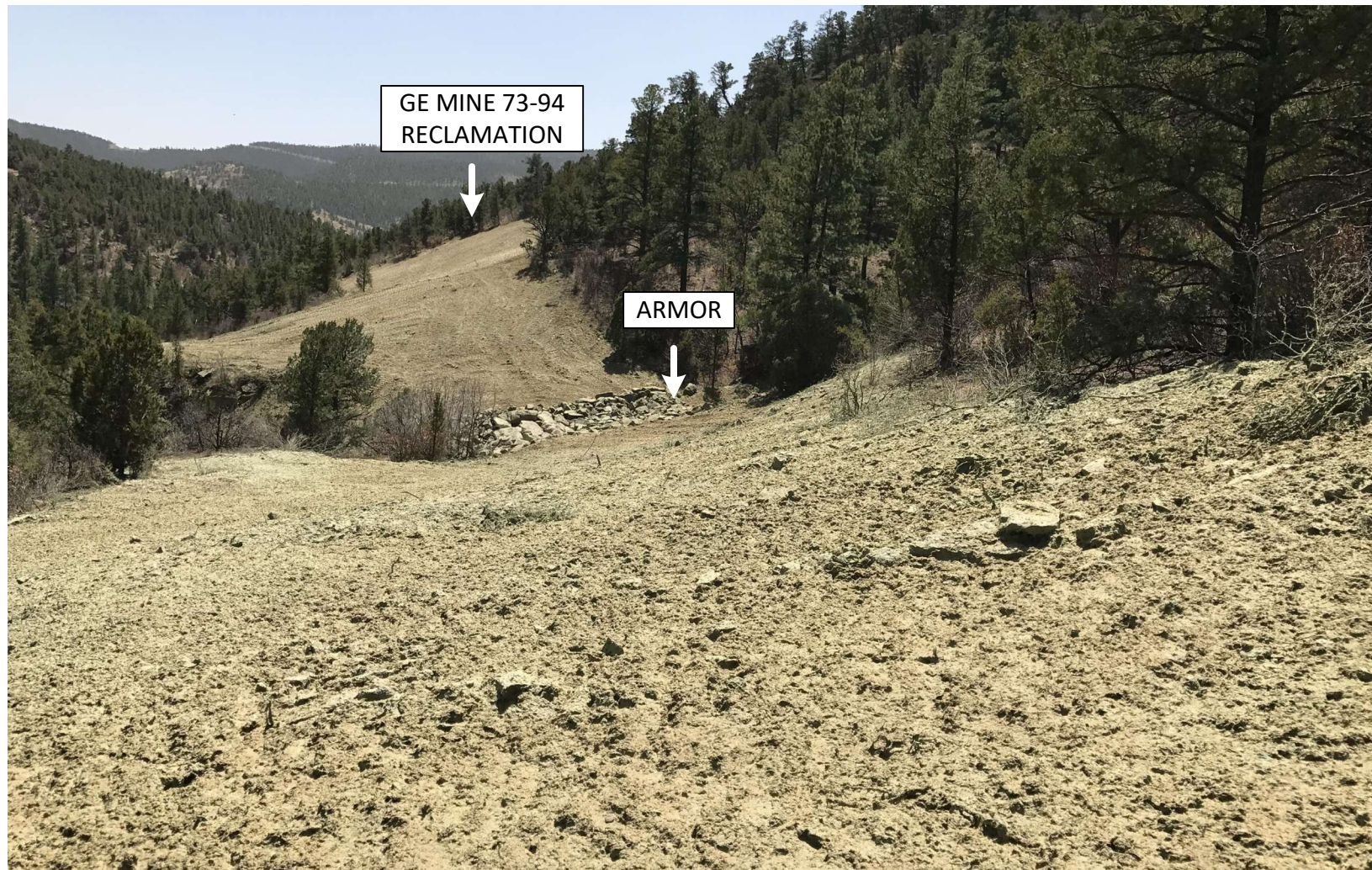
PHOTO 7 : FACING SOUTH TOWARD THE GOLDEN EAGLE (GE) MINE 73-94 WELL PAD RECLAMATION. THE MAIN ACCESS ROAD NORTH OF THE GE 73-94 WAS RECONTOURED TO MATCH THE SURROUNDING TERRAIN. GRADING TECHNIQUES WERE INSTALLED ON THE CONTOUR TO PROMOTE GROUND INFILTRATION FROM RUN OFF. THE EARTH DISTURBANCE WAS STABILIZED BY HYDRO-SEEDING USING AN APPROVED HILL RANCH SEED MIX TO PROMOTE THE ESTABLISHMENT OF VEGETATION. ARMOR WAS PLACED IN THE ARROYO FOR EROSION CONTROLL DURING RUN OFF EVENTS.
