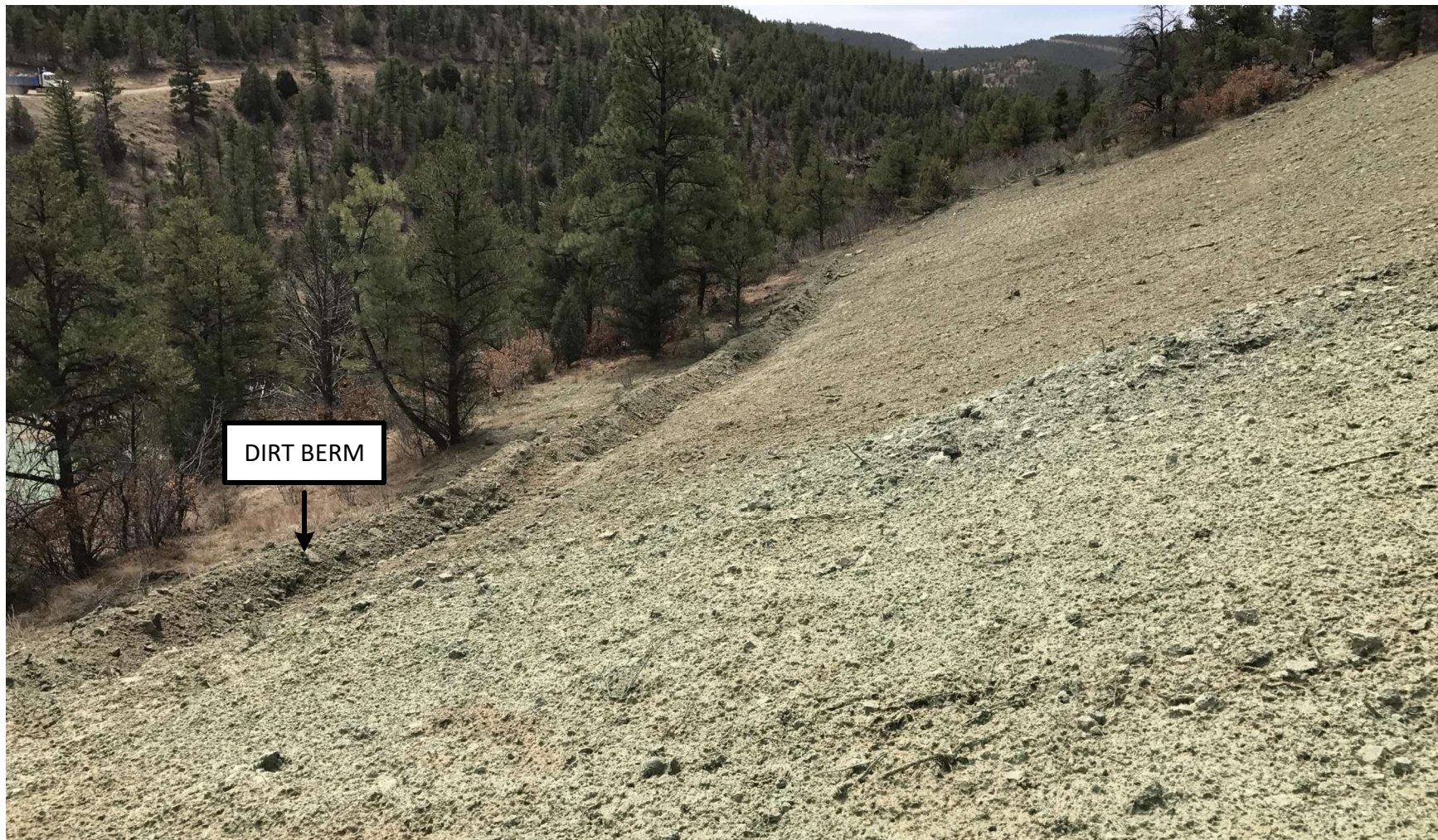
PHOTO 2 : GOLDEN EAGLE MINE 73-94 RECLAMATION. WELL PAD WAS RECONTOURED TO MATCH THE SURROUNDING TERRAIN. GRADING TECHNIQUES WERE INSTALLED ON THE CONTOUR TO PROMOTE GROUND INFILTRATION AND PREPARE THE SOIL FOR SEEDING. THE EARTH DISTURBANCE WAS STABILIZED BY HYDRO-SEEDING USING AN APPROVED HILL RANCH SEED MIX TO PROMOTE THE ESTABLISHMENT OF VEGETATION. THE TOP SOIL STOCKPILE WAS UTILIZED DURING RECLAMATION ACTIVITIES. A DIRT BERM WAS INSTALLED DOWN GRADIENT OF THE PROJECT TO PROVIDE PERIMETER SEDIMENT CONTROL FOR THE WELL PAD. ALL WEEDS WERE SCRAPED UP AND BURIED IN THE SOIL DURING THE RECLAMATION ACTIVITIES. ALL RECLAMATION PROJECTS WILL BE INCORPORATED INTO TIMBER CREEK'S WEED MANAGEMENT PLAN. ALL THE LOCATION SIGN AND POSTS WERE REMOVED FROM LOCATION.
