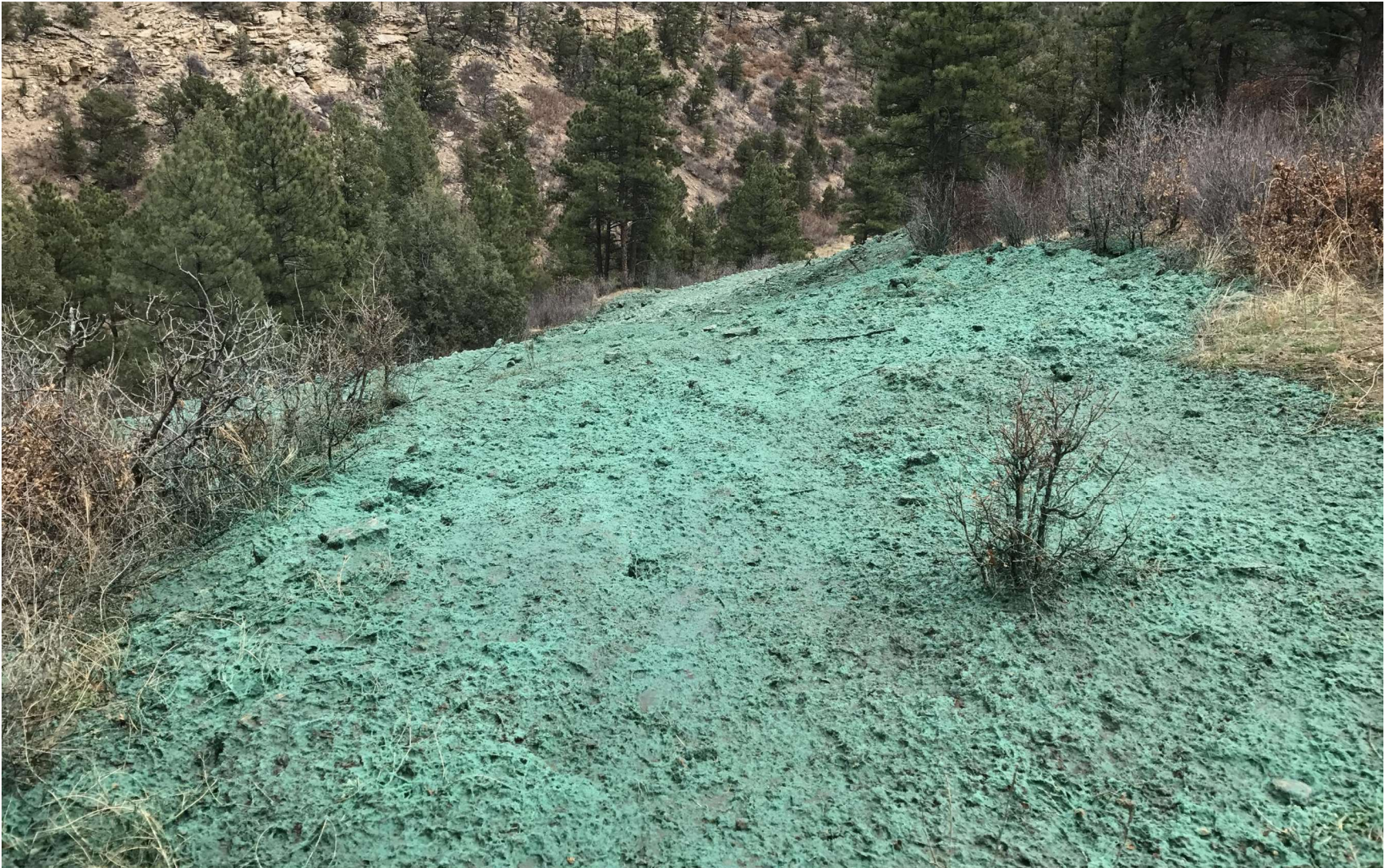
PHOTO 14 : ACCESS ROAD RECLAMATION NORTHEAST OF THE PRODUCING WELL GOLDEN EAGLE 20-09 API # 071-08803. THE ACCESS ROAD WAS RECONTOURED TO MATCH THE SURROUNDING TERRAIN. SOIL ROUGHENING WAS USED TO PROMOTE GROUND INFILTRATION AND PREPARE THE SOIL FOR SEEDING. THE EARTH DISTURBANCE WAS STABILIZED BY HYDRO-SEEDING USING AN APPROVED HILL RANCH SEED MIX TO PROMOTE THE ESTABLISHMENT OF VEGETATION.
