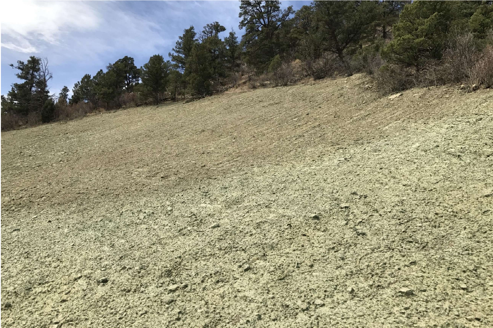
PHOTO 3 : GOLDEN EAGLE MINE 73-94 RECLAMATION. THE WELL PAD WAS RECONTOURED TO MATCH THE SURROUNDING TERRAIN. GRADING TECHNIQUES WERE INSTALLED ON THE CONTOUR TO PROMOTE GROUND INFILTRATION AND PREPARE THE SOIL FOR SEEDING. THE EARTH DISTURBANCE WAS STABILIZED BY HYDRO-SEEDING USING AN APPROVED HILL RANCH SEED MIX TO PROMOTE THE ESTABLISHMENT OF VEGETATION. ALL WEEDS WERE SCRAPED UP AND BURIED IN THE SOIL DURING THE RECLAMATION ACTIVITIES. ALL RECLAMATION PROJECTS WILL BE INCORPERATED INTO TIMBER CREEK'S WEED MANAGEMENT PLAN.
