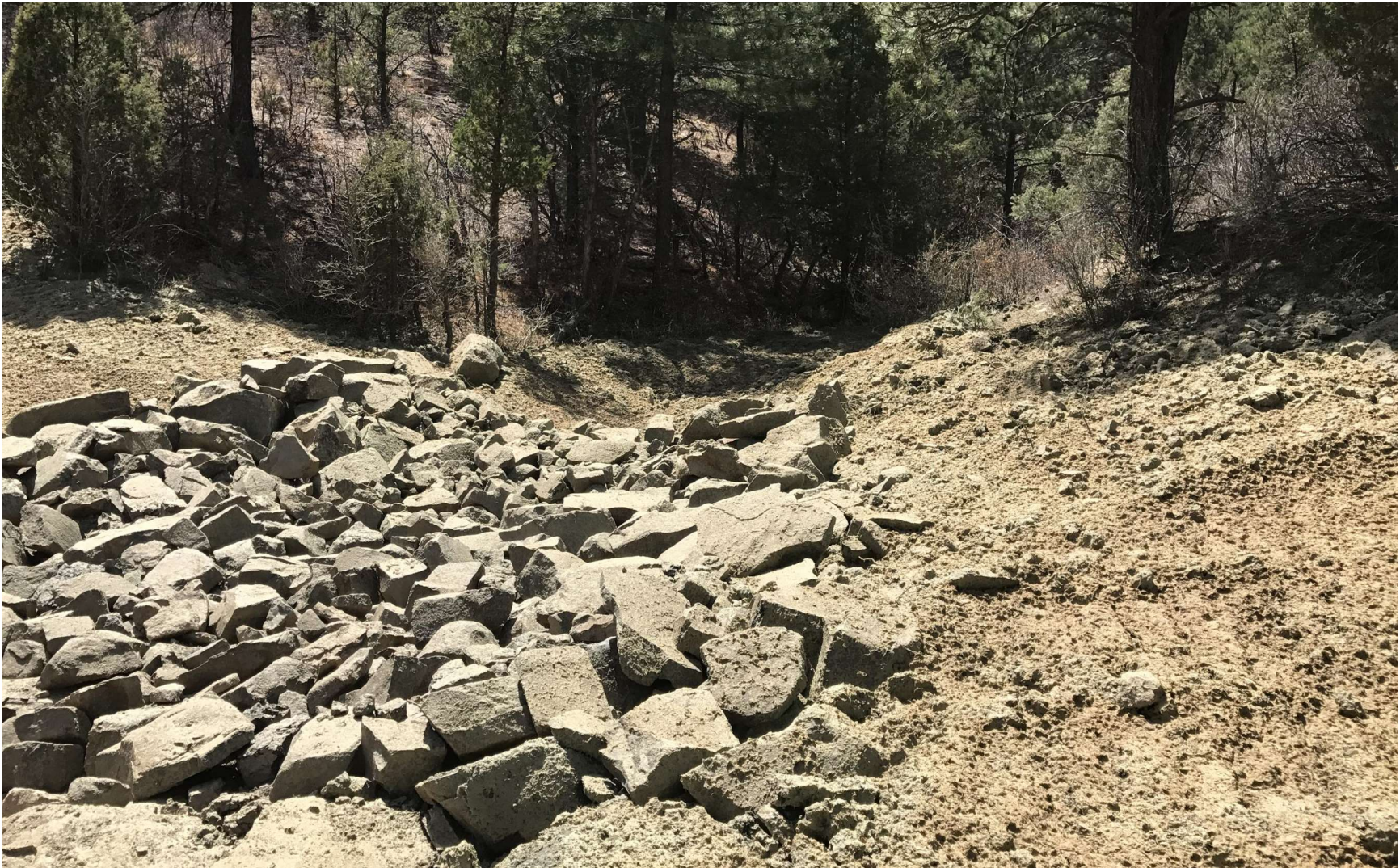
PHOTO 8: ARMOR WAS PLACED IN THE ARROYO FOR EROSION CONTROLL DURING RUN OFF EVENTS.
