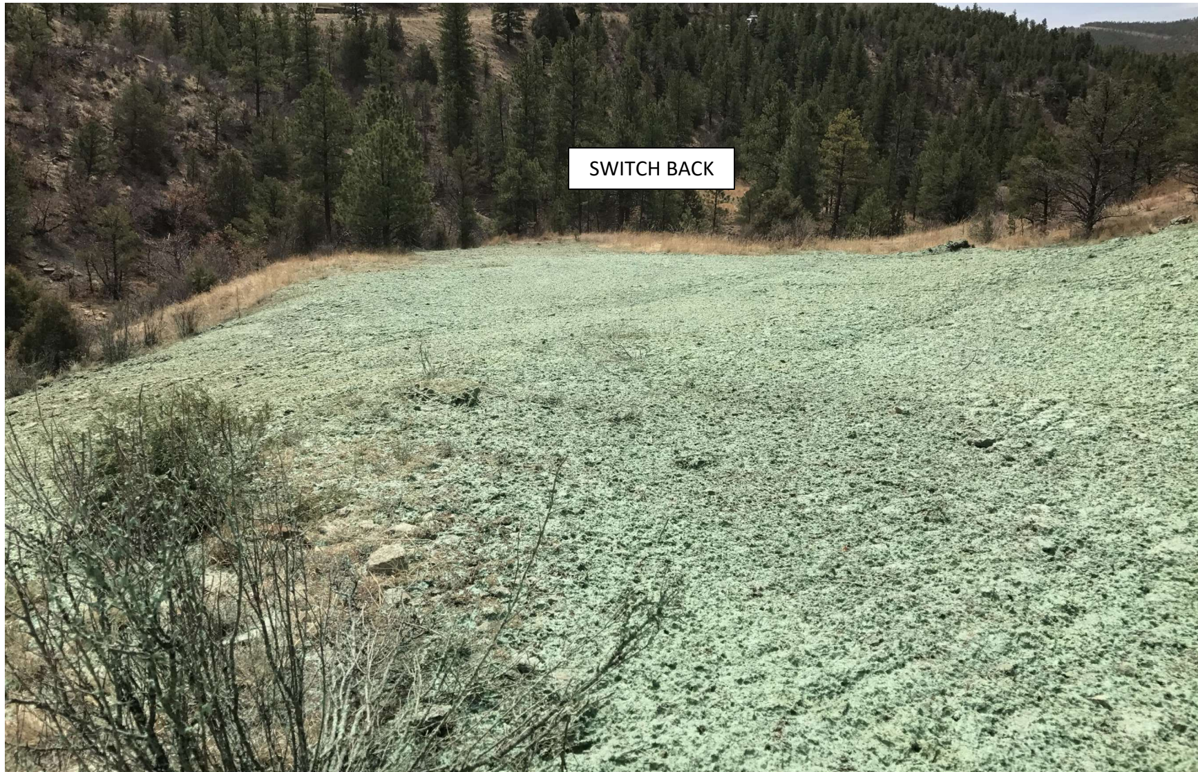
PHOTO 5 : FACING SOUTH ALONG THE MAIN ACCESS ROAD EAST OF THE GOLDEN EAGLE MINE 73-94 WELL PAD. THE MAIN ACCESS ROAD WAS RECONTOURED TO MATCH THE SURROUNDING TERRAIN. GRADING TECHNIQUES WERE INSTALLED ON THE CONTOUR TO PROMOTE GROUND INFILTRATION AND PREPARE THE SOIL FOR SEEDING. THE EARTH DISTURBANCE WAS STABILIZED BY HYDRO-SEEDING USING AN APPROVED HILL RANCH SEED MIX TO PROMOTE THE ESTABLISHMENT OF VEGETATION.
