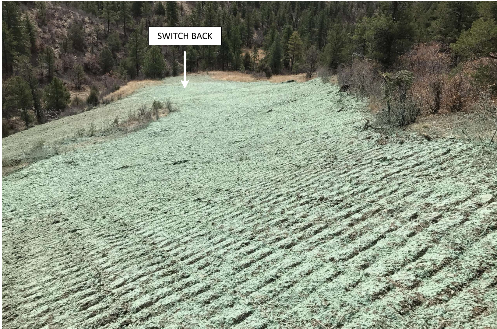
PHOTO 4 : FACING SOUTH ALONG THE MAIN ACCESS ROAD EAST OF THE GOLDEN EAGLE MINE 73-94 WELL PAD. THE MAIN ACCESS ROAD WAS RECONTOURED TO MATCH THE SURROUNDING TERRAIN. GRADING TECHNIQUES WERE INSTALLED ON THE CONTOUR TO PROMOTE GROUND INFILTRATION AND PREPARE THE SOIL FOR SEEDING. THE EARTH DISTURBANCE WAS STABILIZED BY HYDRO-SEEDING USING AN APPROVED HILL RANCH SEED MIX TO PROMOTE THE ESTABLISHMENT OF VEGETATION.
