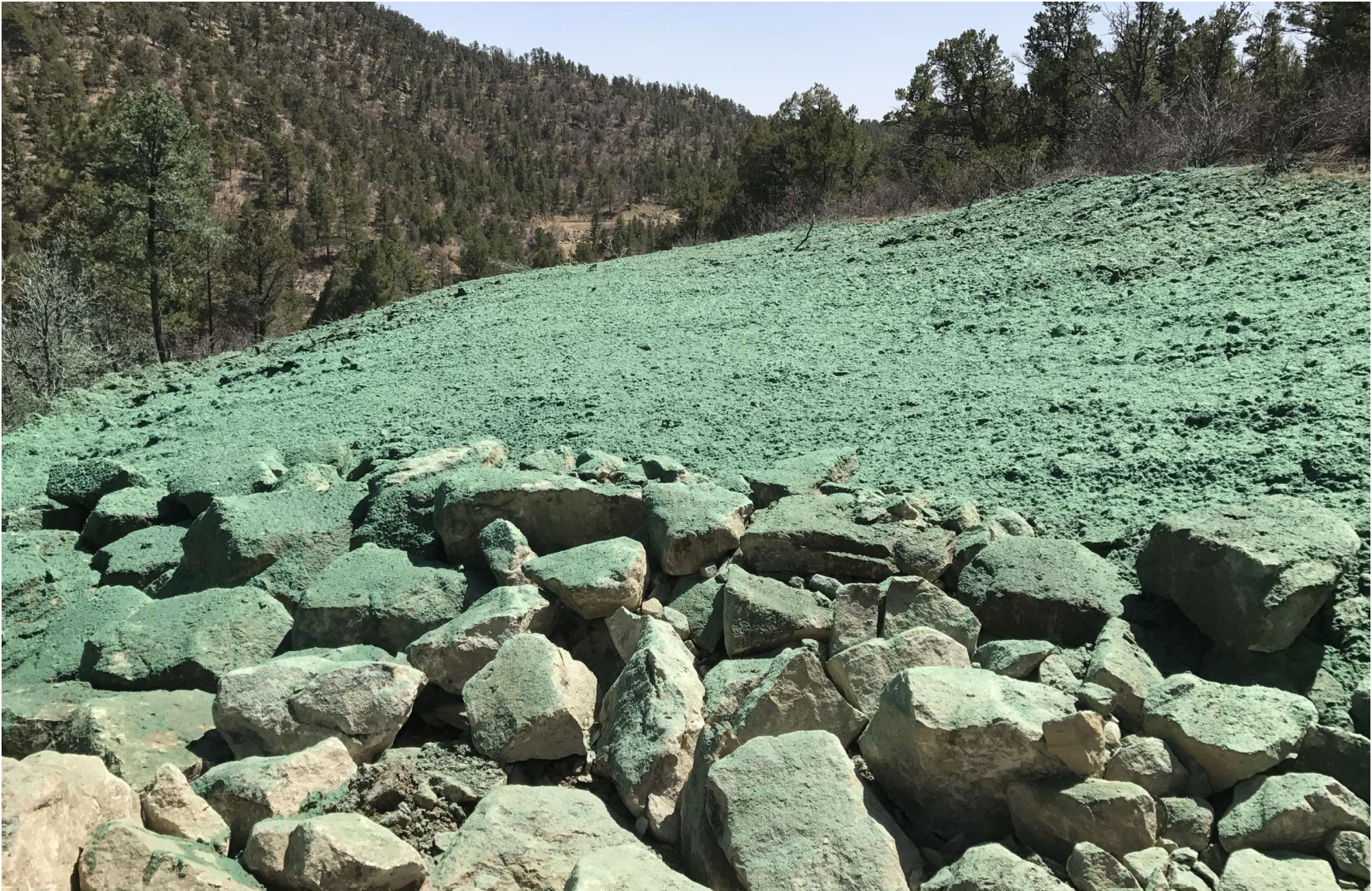
PHOTO 10 : FACING SOUTH, THE MAIN ACCESS ROAD NORTH OF THE GE 73-94 WAS RECONTOURED TO MATCH THE SURROUNDING TERRAIN. GRADING TECHNIQUES WERE INSTALLED ON THE CONTOUR TO PROMOTE GROUND INFILTRATION AND PREPARE THE SOIL FOR SEEDING. THE EARTH DISTURBANCE WAS STABILIZED BY HYDRO-SEEDING USING AN APPROVED HILL RANCH SEED MIX TO PROMOTE THE ESTABLISHMENT OF VEGETATION. ARMOR WAS PLACED IN THE ARROYO FOR EROSION CONTROLL DURING RUN OFF EVENTS.
