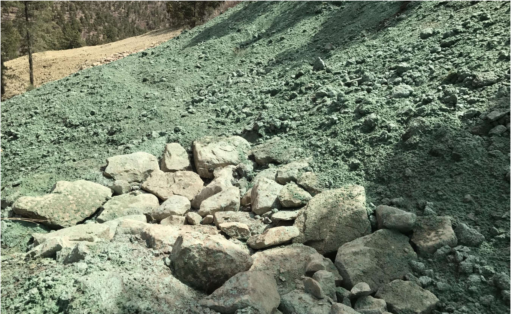
PHOTO 12 : FACING SOUTH, THE MAIN ACCESS ROAD BELOW THE PRODUCING WELL GOLDEN EAGLE 20-09 API # 071-08803 WAS RECONTOURED TO MATCH THE SURROUNDING TERRAIN. SOIL ROUGHENING WAS USED TO PROMOTE GROUND INFILTRATION AND PREPARE THE SOIL FOR SEEDING. THE EARTH DISTURBANCE WAS STABILIZED BY HYDRO-SEEDING USING AN APPROVED HILL RANCH SEED MIX TO PROMOTE THE ESTABLISHMENT OF VEGETATION. ARMOR WAS PLACED WHERE RUN OFF WILL DISCHARGE FOR EROSION CONTROLL.
