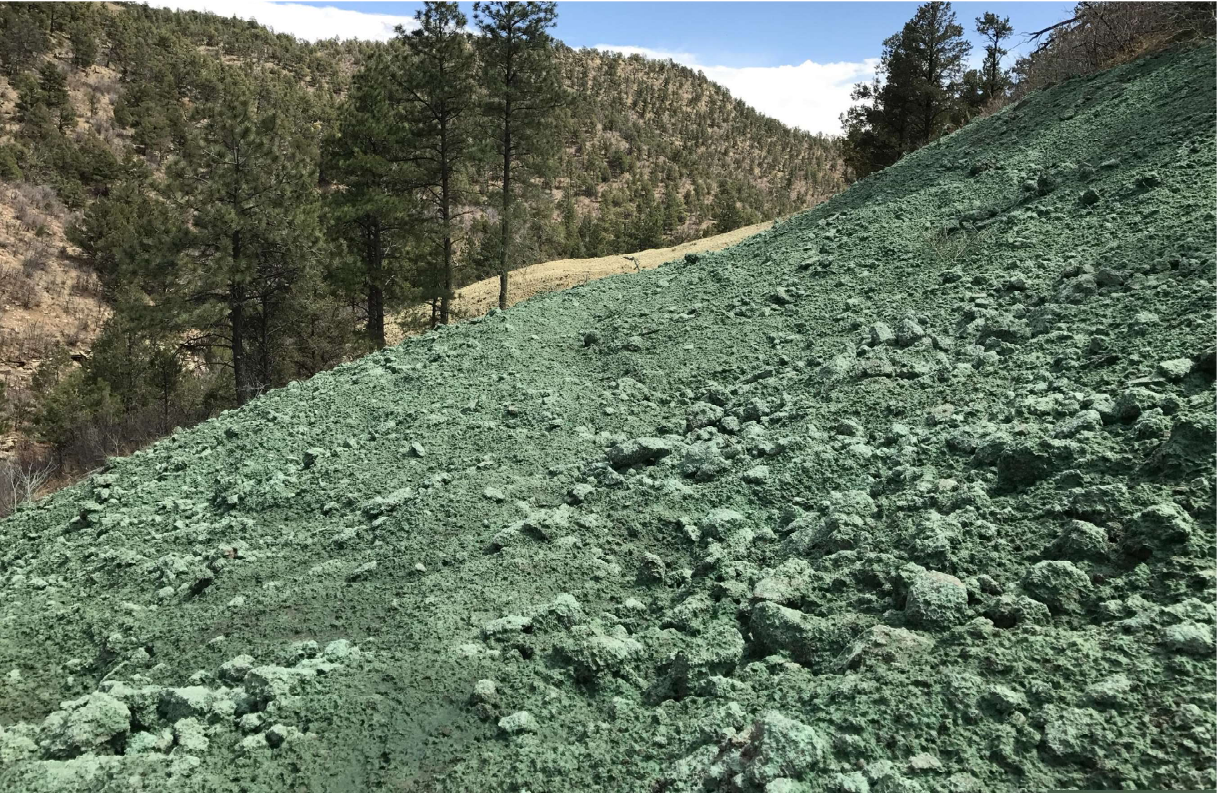
PHOTO 11 : FACING SOUTH, THE MAIN ACCESS ROAD BELOW THE PRODUCING WELL GOLDEN EAGLE 20-09 API # 071-08803 WAS RECONTOURED TO MATCH THE SURROUNDING TERRAIN. SOIL ROUGHENING WAS USED TO PROMOTE GROUND INFILTRATION AND PREPARE THE SOIL FOR SEEDING. THE EARTH DISTURBANCE WAS STABILIZED BY HYDRO-SEEDING USING AN APPROVED HILL RANCH SEED MIX TO PROMOTE THE ESTABLISHMENT OF VEGETATION.
