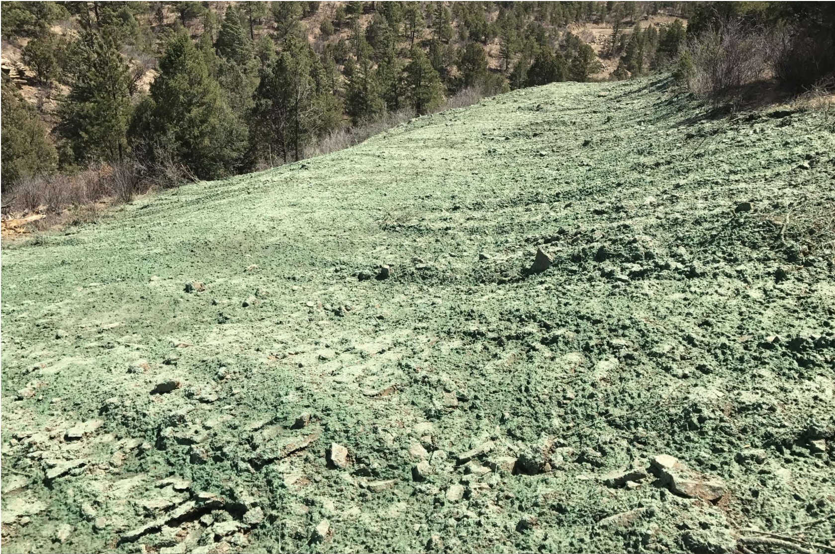
PHOTO 9 : FACING SOUTH, THE MAIN ACCESS ROAD NORTH OF THE GE 73-94 WAS RECONTOURED TO MATCH THE SURROUNDING TERRAIN. GRADING TECHNIQUES WERE INSTALLED ON THE CONTOUR TO PROMOTE GROUND INFILTRATION AND PREPARE THE SOIL FOR SEEDING. THE EARTH DISTURBANCE WAS STABILIZED BY HYDRO-SEEDING USING AN APPROVED HILL RANCH SEED MIX TO PROMOTE THE ESTABLISHMENT OF VEGETATION.
