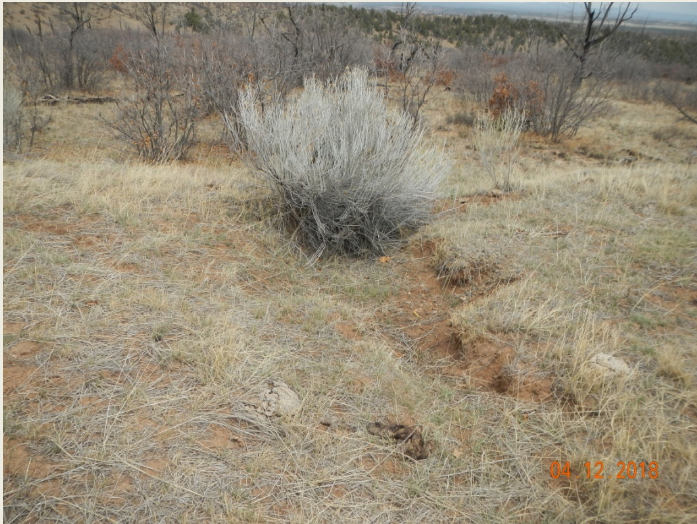
Photo 7. View of head-cut and erosional channel forming within the northeastern portion of the project area.
