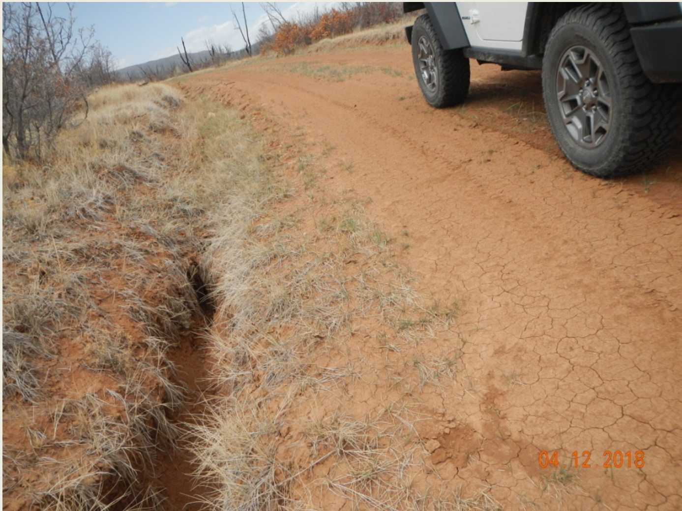
Photo 8. View of head-cut and erosional channel forming along the access road, up to 1.5 feet deep.
