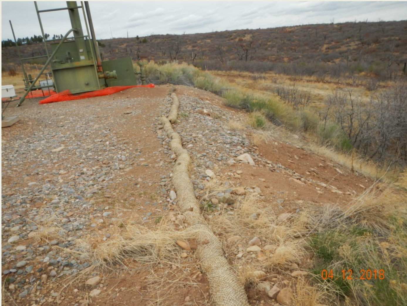
Photo 4. View of wattles on the eastern edge of the working area. This is a temporary stormwater control and will need careful monitoring and maintenance as needed.
