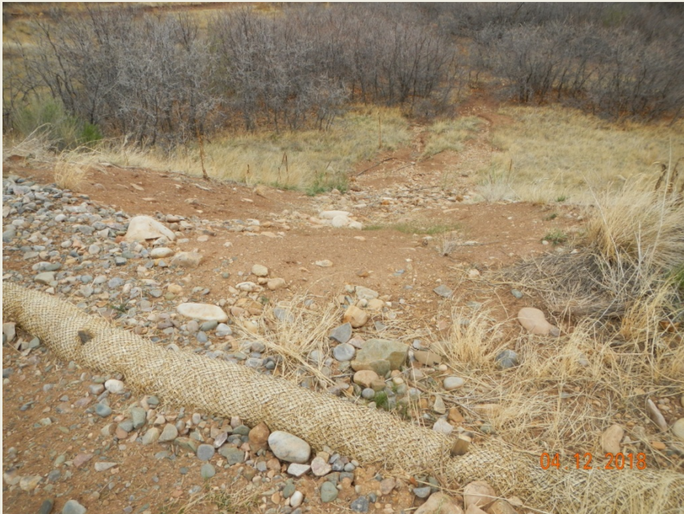
Photo 5. View of area in eastern project area with exposed soils, appears to be disturbed for erosion control and needs re-seeding/stabilization measures.
