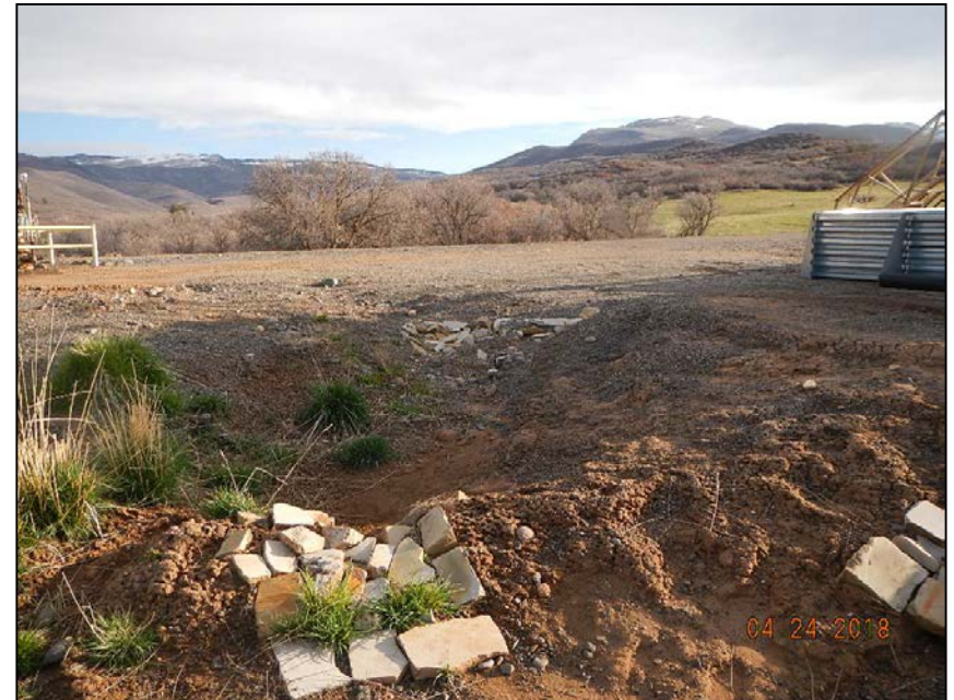
Photo 2. Erosion controls on South edge of location.
