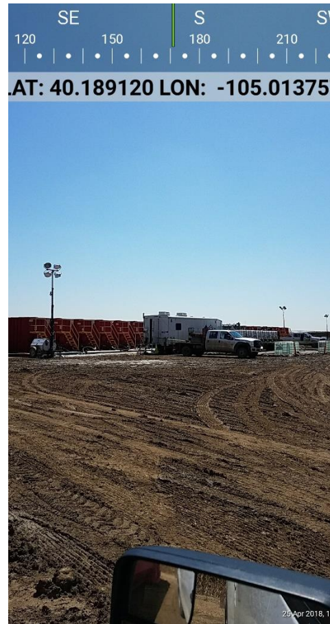
Photo 2 Water Tanks and Lights
