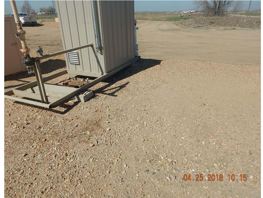
Photo 4: Risers removed
