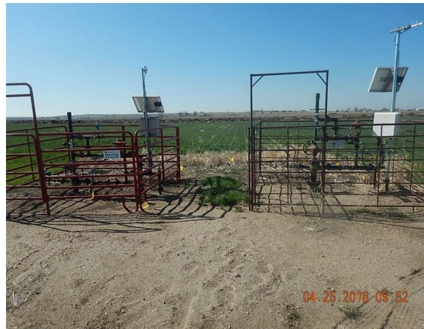
Photo 2: Wellheads, looking S. Bradenhead plumbed to surface.
