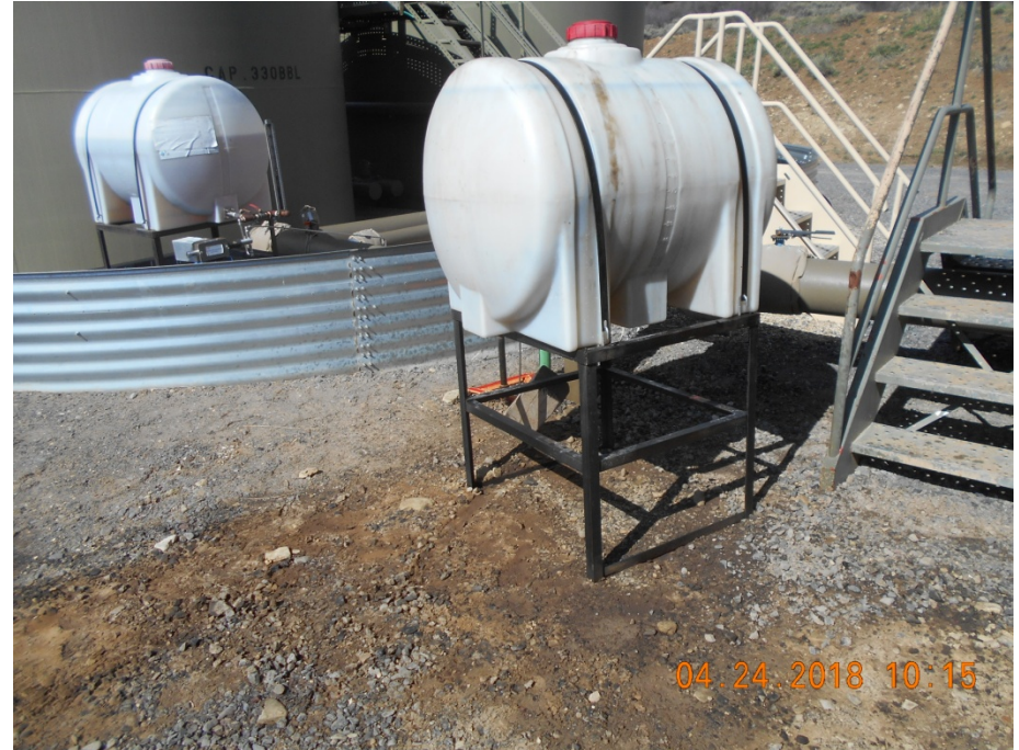
Chemical storage with no secondary containment.
