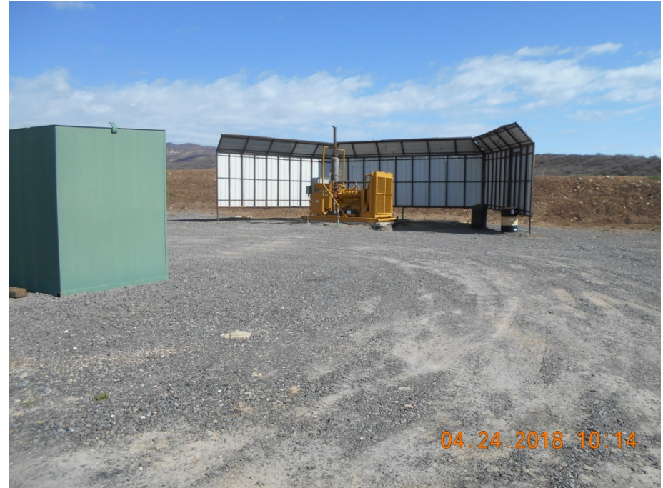
Generator with sound wall
