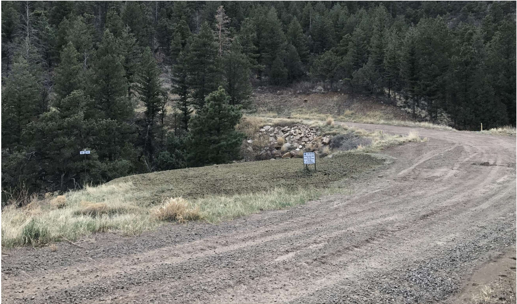
PHOTO 2: THE GRAVEL ON THE WELL PAD WAS REMOVED. THE EARTH DISTURBANCE WAS HYDRO-SEEDED WITH AN APPROVED HILL RANCH SEED MIX TO PROMOTE THE ESTABLISHMENT OF VEGETATION.
