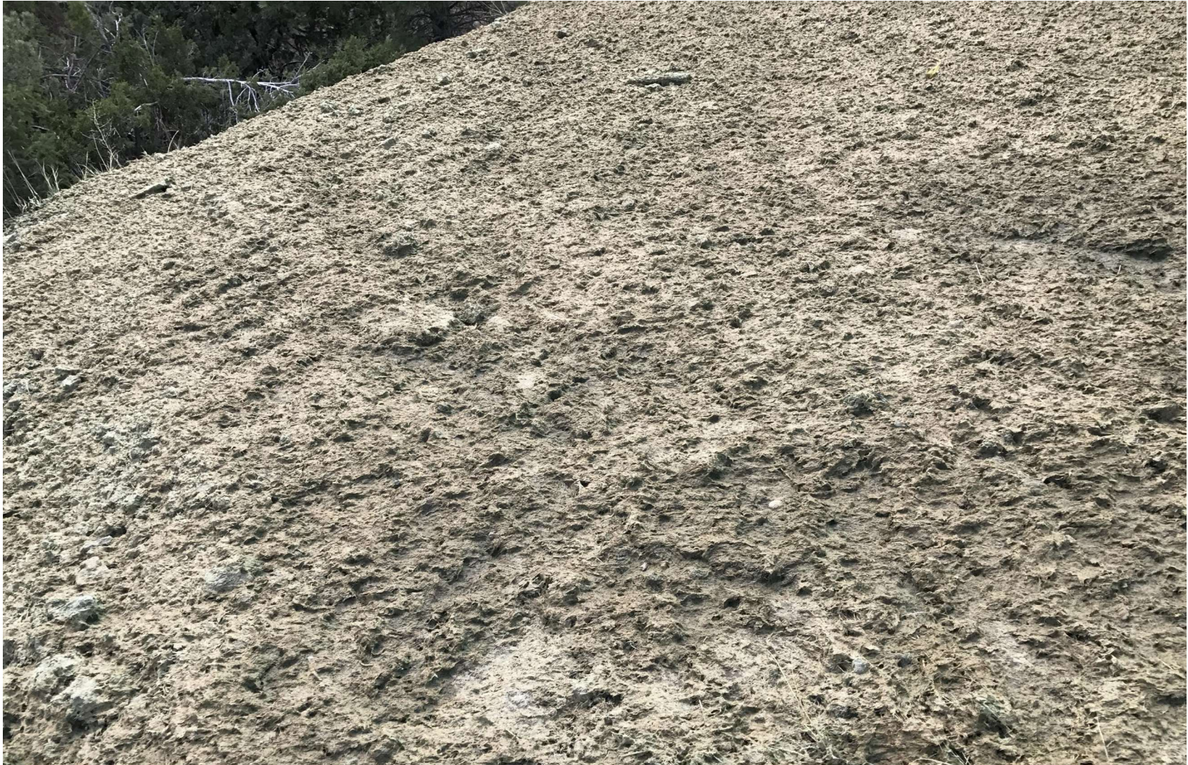
PHOTO 3: THE GRAVEL ON THE WELL PAD WAS REMOVED. SOIL WAS DELIVERED TO RECONTOUR THE PAD WHERE THE GRAVEL WAS REMOVED. THE EARTH DISTURBANCE WAS HYDRO-SEEDED WITH AN APPROVED HILL RANCH SEED MIX TO PROMOTE THE ESTABLISHMENT OF VEGETATION.
