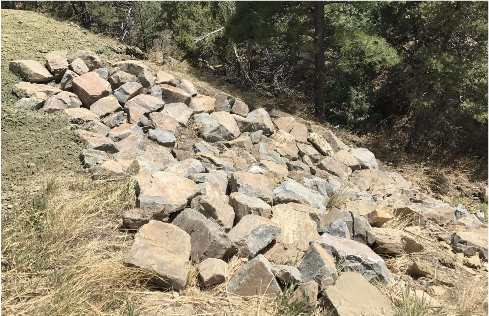
PHOTO 5: LOCATION WHERE STORMWATER DISCHARGES INTO RAVINE. THIS AREA ON THE SOUTHWEST CORNER OF THE PAD WAS ARMORED FOR LONG TERM EROSION CONTROL.
