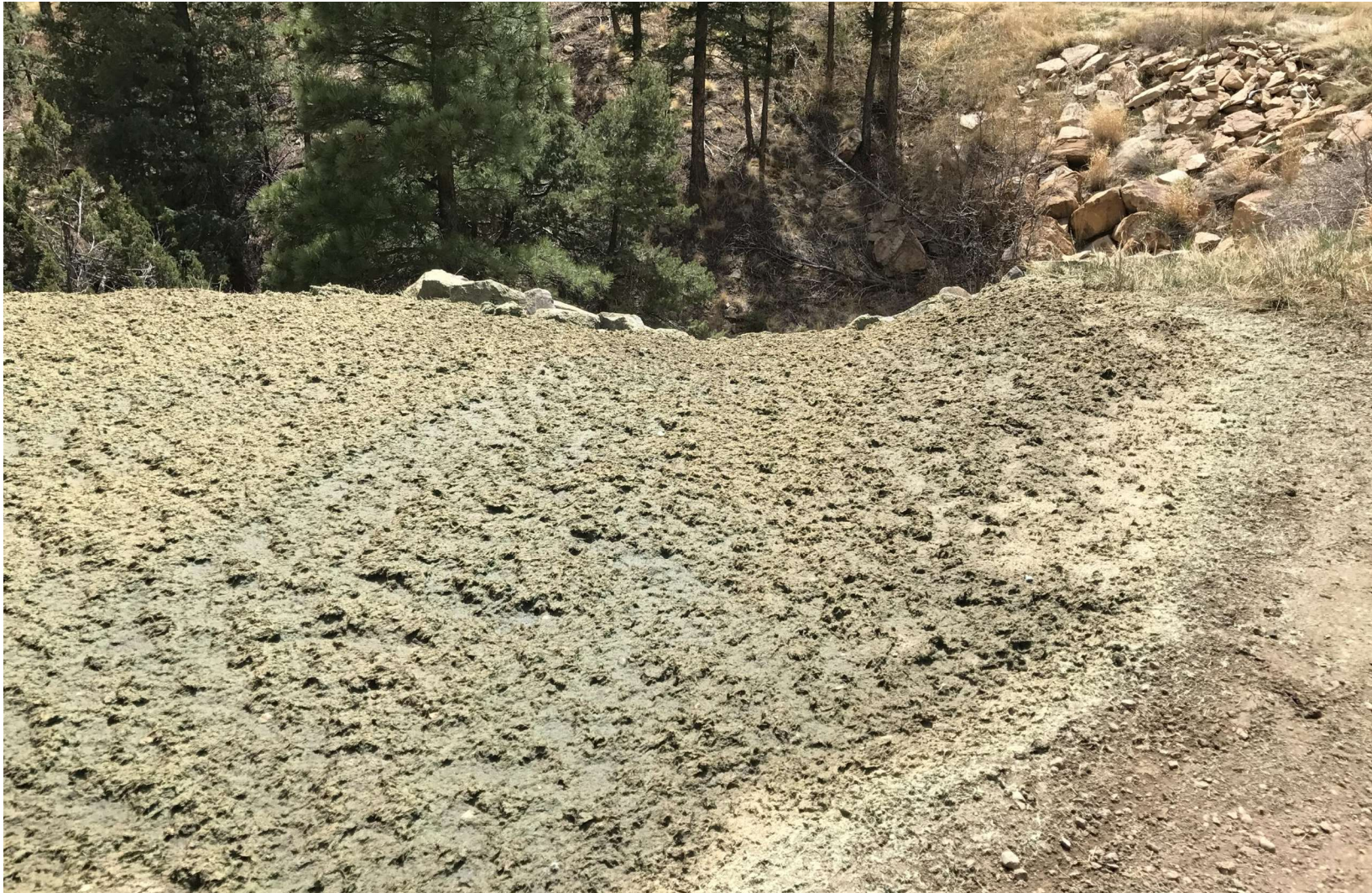
PHOTO 4: LOCATION WHERE STORMWATER DISCHARGES INTO RAVINE. THIS AREA ON THE SOUTHWEST CORNER OF THE PAD WAS SWELLED OUT TO RECEIVE RUN OFF FROM THE ACCESS ROAD AS SHEET FLOW.
