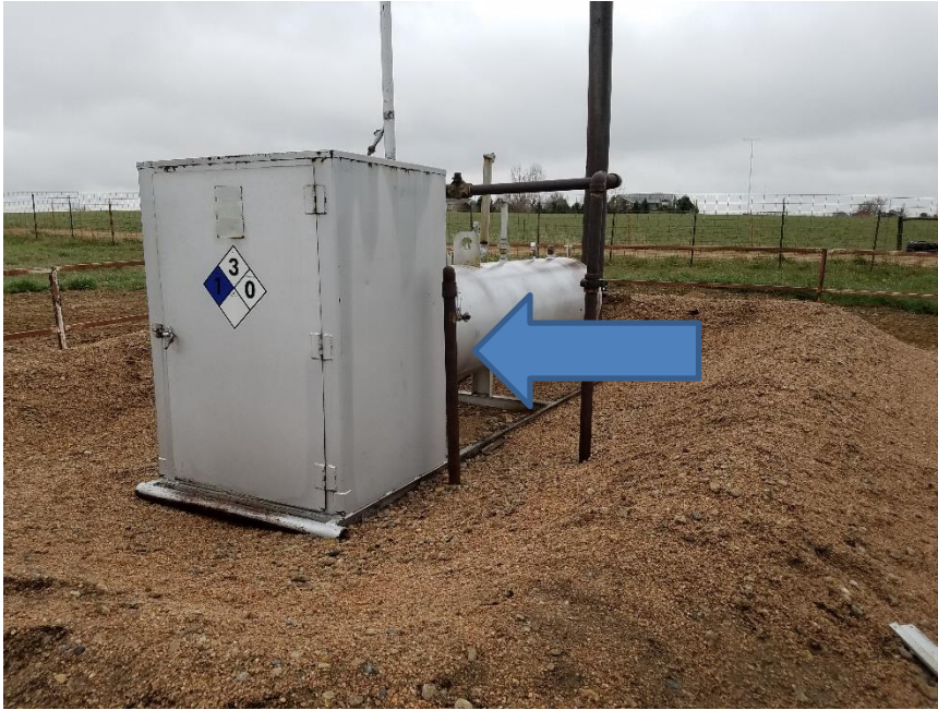
Photo 3. Unmarked riser
