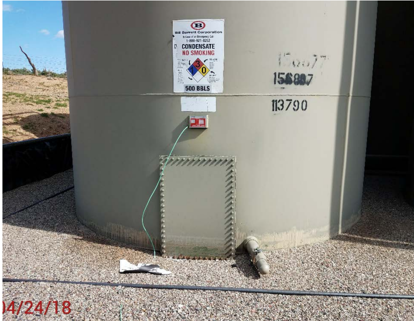
Location photo # 3 Missing/ wrong tank information
