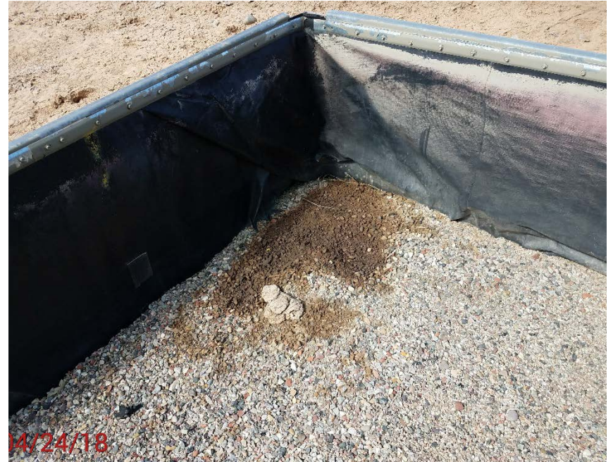
Location photo # 6 staining inside tank containment
