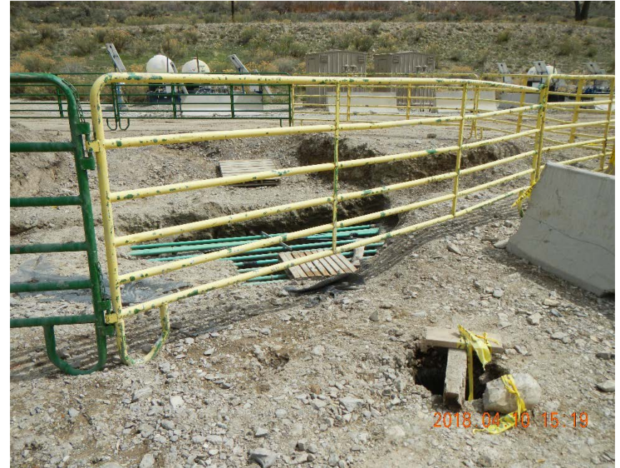
Looking east. Area excavated with hydrovac. Pipeline corridor with multiple pipelines difficult excavation.
