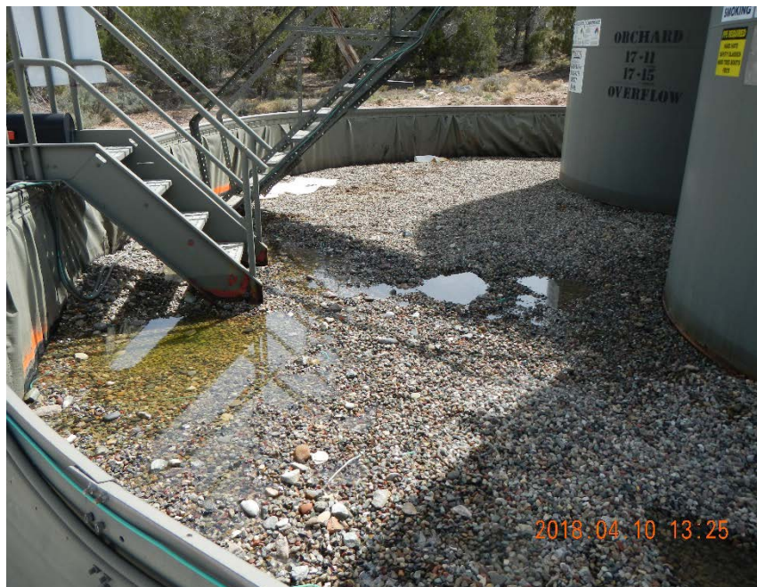
North side of tank battery. Caerus conducted a hydrostatic test to determine if liner was compromised. Approximately 5 holes were detected on the north side near the external wall.
