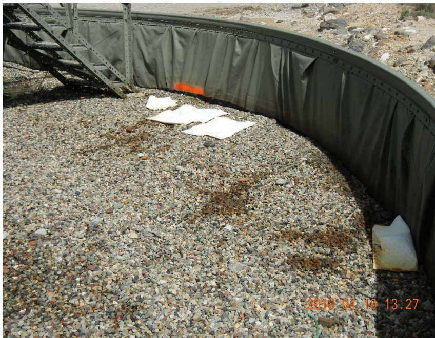
North side of the tank battery. Absorbent pads. According to Caerus, spilled produced water had very little HCs.
