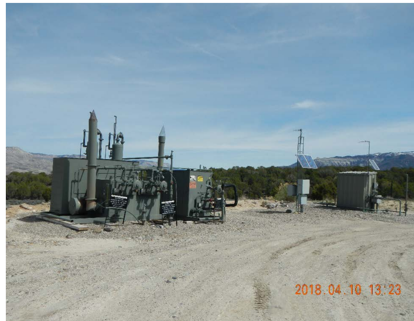
Looking north. Separators and meter house near the entrance.
