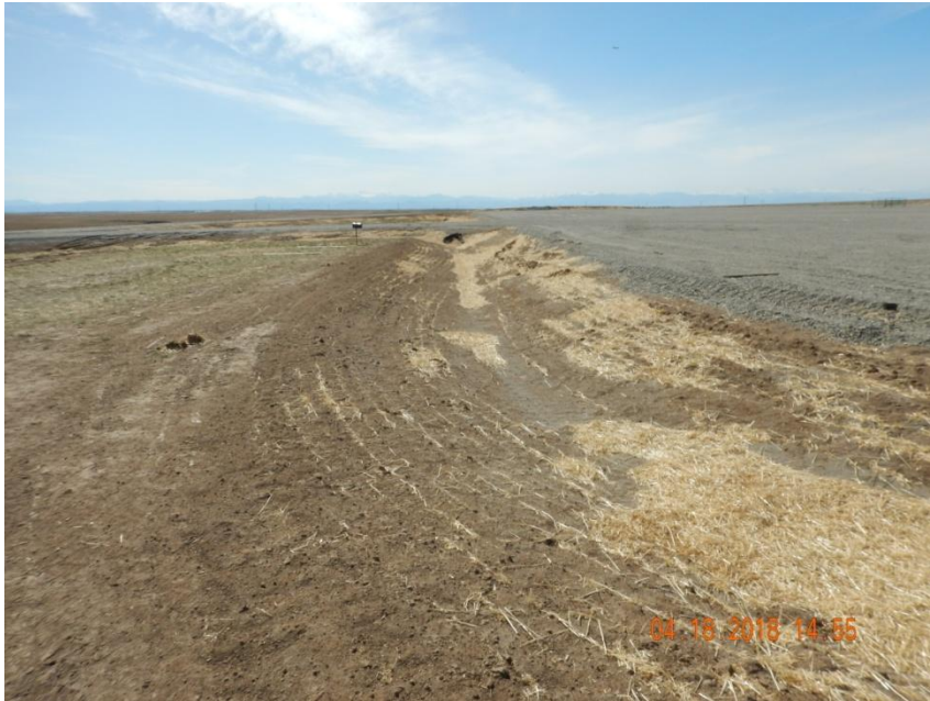
Photo 1. Photo taken from southeastern perimeter of location, facing West. Ditch and berm BMP has been installed along the entire well pad perimeter of the location which is directed to stabilized outlets. Appears the ditch and berm BMP has been seeded and straw crimped. Straw crimping does not appear to have stayed crimped as loose material was observed throughout. Well pad and access road has been stabilized with gravel.
