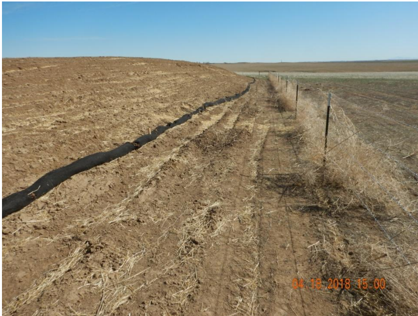
Photo 5. Photo taken from the southwestern location, facing South. Topsoil stockpile appears to be temporarily stabilized by equipment tracking. Topsoil has been seeded and straw mulched. Straw crimping does not appear to have stayed crimped.
