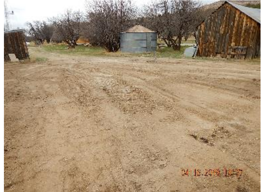
Photo 4: Tank battery overview.
