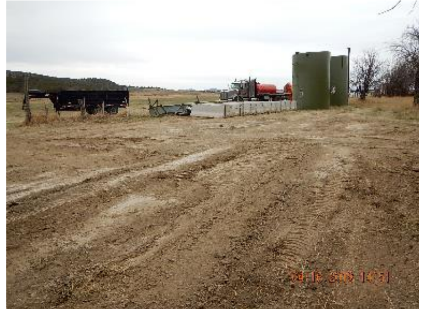
Photo 10: Doerfer 2 well area overview.
