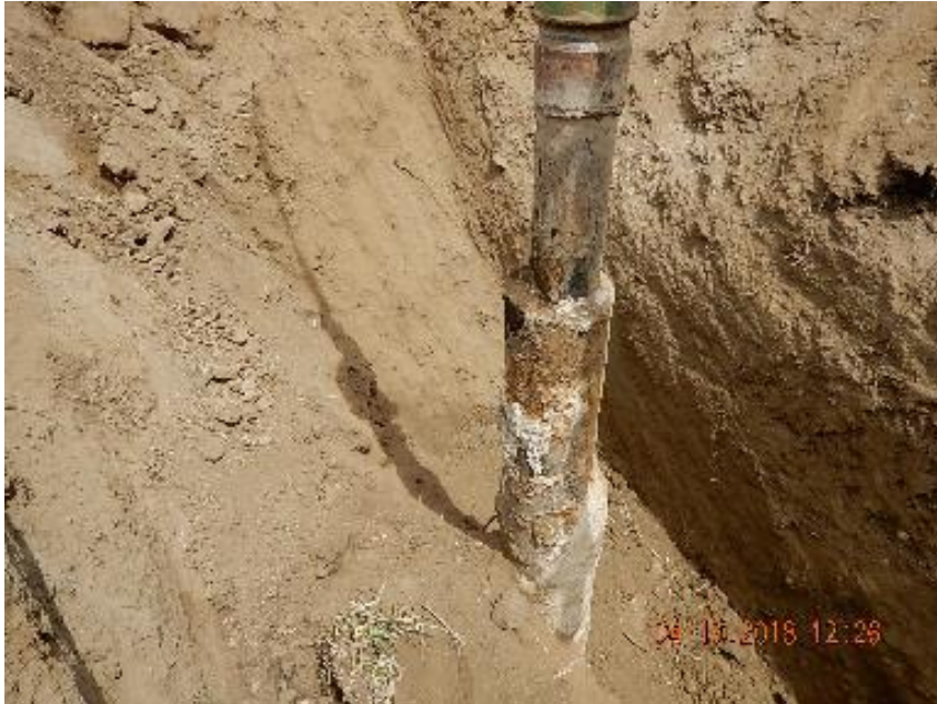
Photo 3: Excavated wellhead casing..
