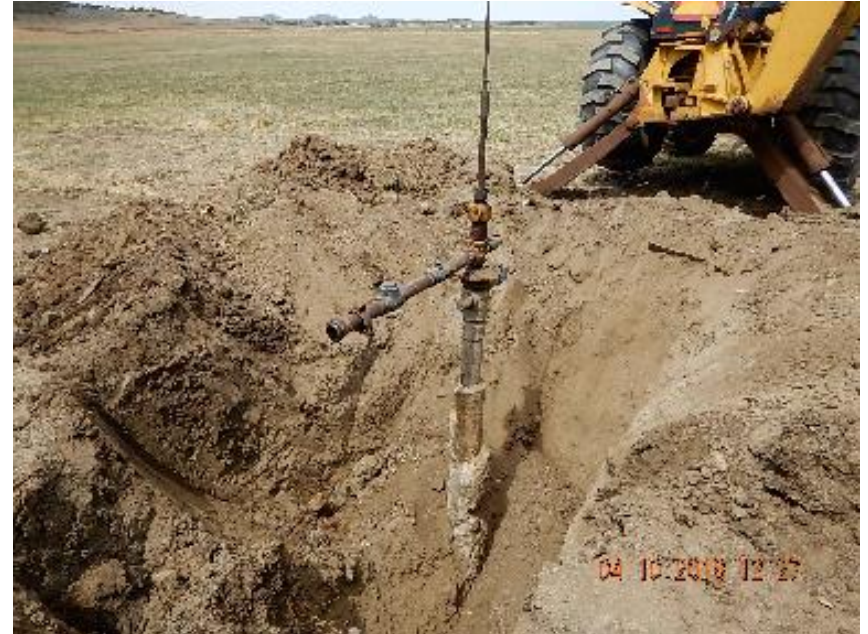
Photo 4: Excavated wellhead casing.
