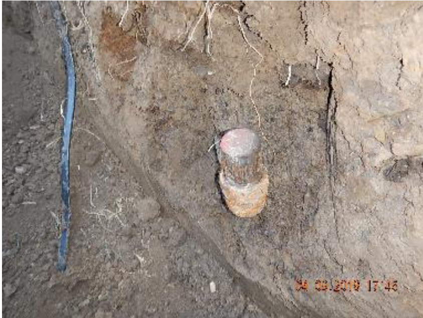
Photo 9: Flow line from Doerfer 1-5 to Doerfer 2 capped with 2" bull plug.
