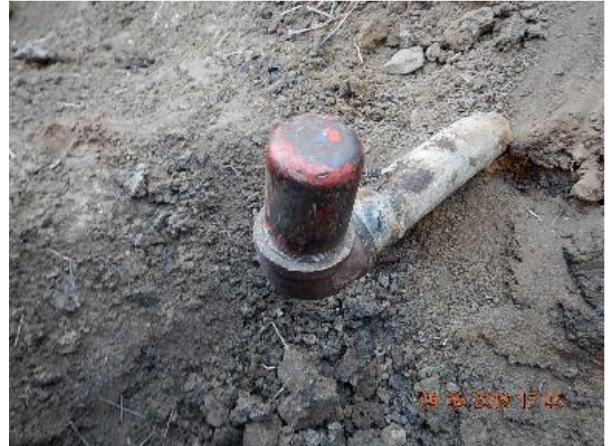
Photo 10: Flow line from Doerfer 2 to tank battery riser capped with 2" bull plug.
