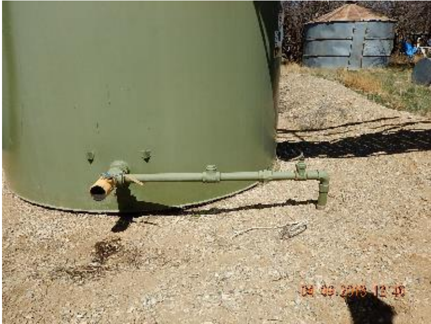
Photo 7: Riser at tank.
