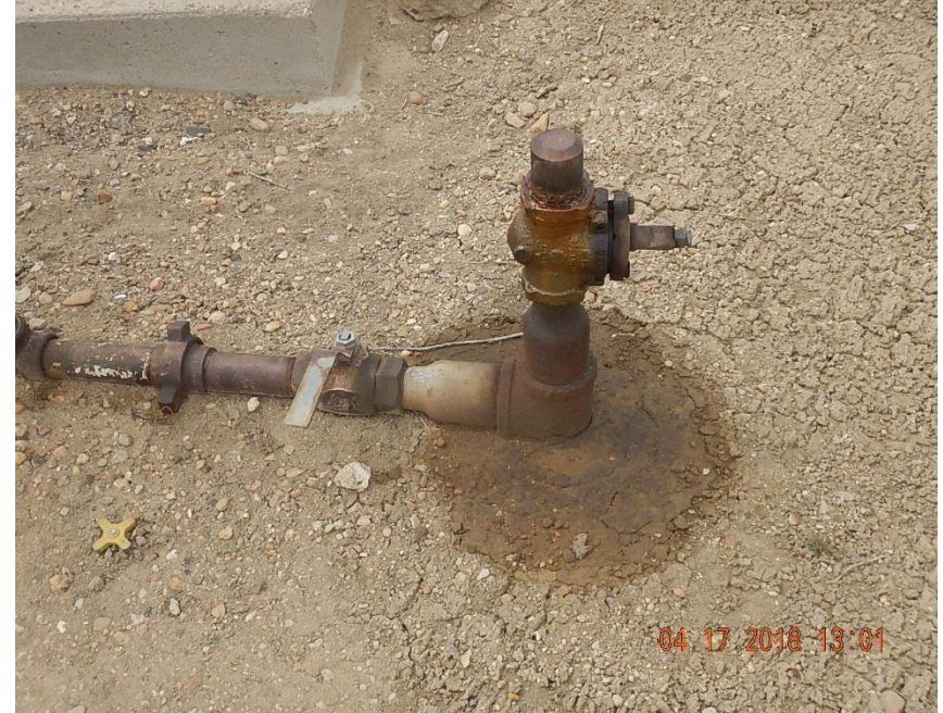
Leaking flowline valve and stained soils
