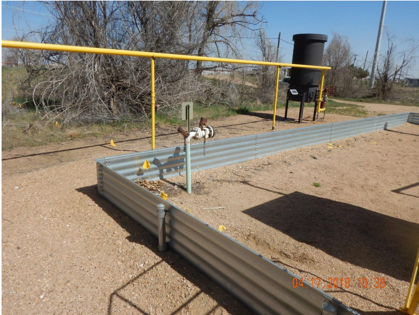
Photo 1: Photo taken from the northern half of Extraction's Brantner tank battery. Photo shows abandoned riser remaining on location.
