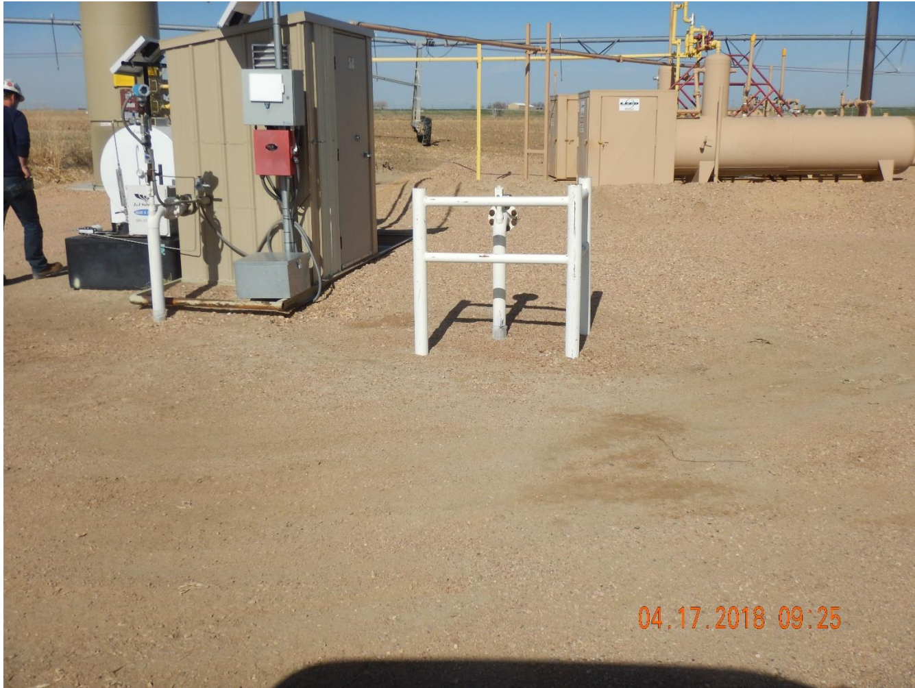
Photo 1: Photo taken from the western half of Noble's Foe tank battery. Photo shows abandoned riser remaining on location.
