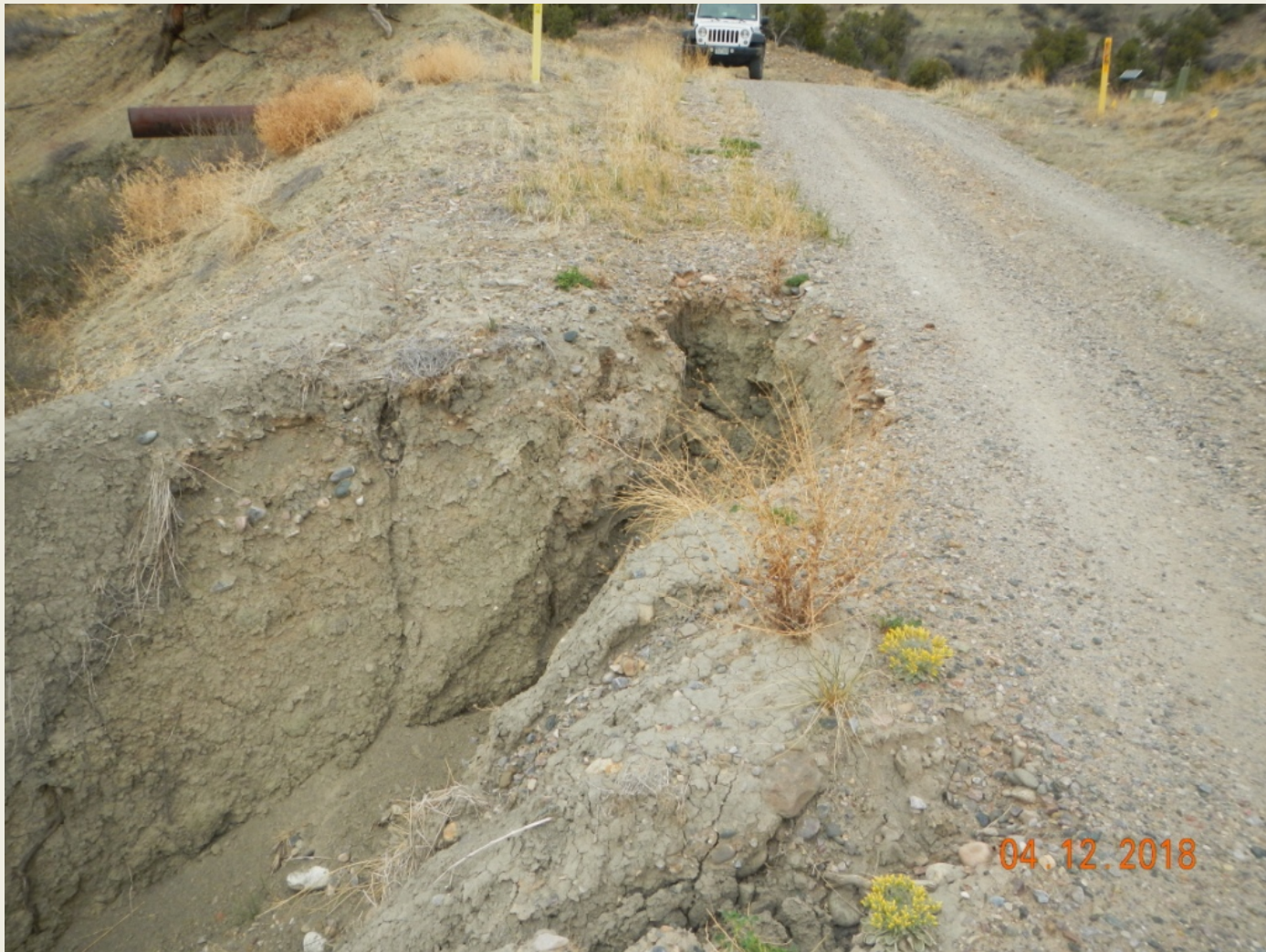
Photo 4. View of erosional channel up to 4 feet deep along the roadside near the entrance to the well pad entrance.
