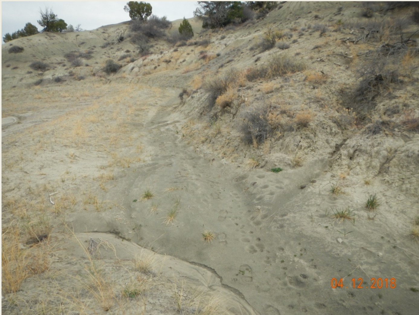
Photo 3. View of the northeastern project area from the eastern edge facing northwestward. Diversion channel is full of sediment and cut-slopes are eroding in the northern and northeastern project area. Revegetation is progressing on berms.
