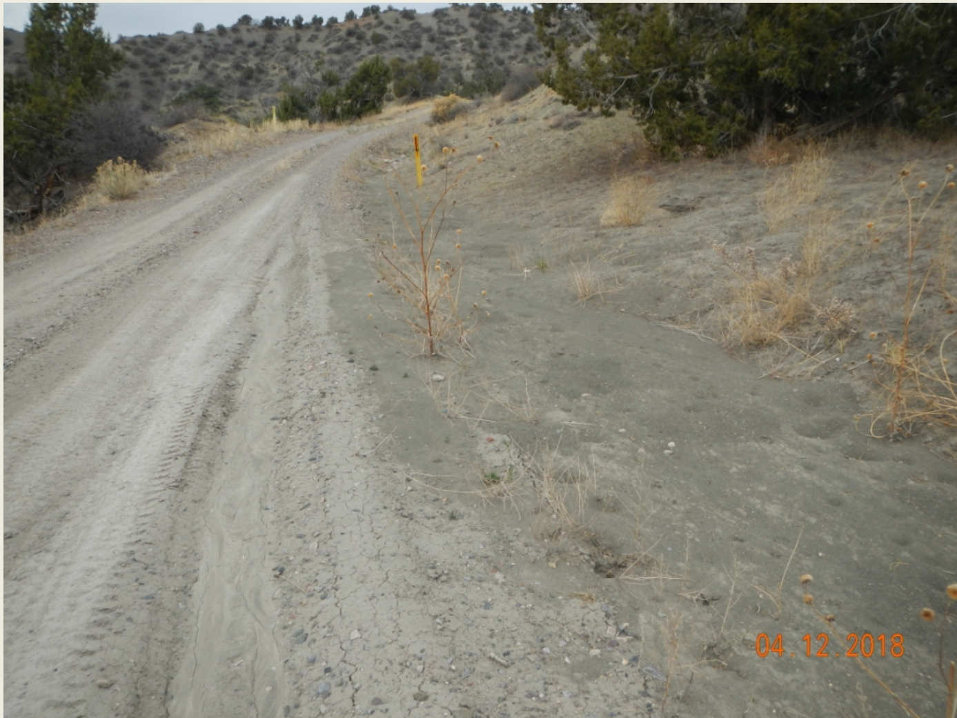
Photo 7. View of area where roadside drainage is full of sediment. Sediment controls are needed here.
