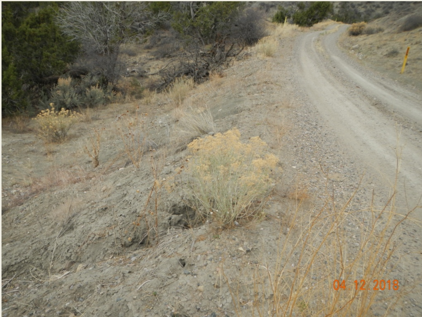
Photo 8. View of erosional rilling along the access road, needs stabilization.
