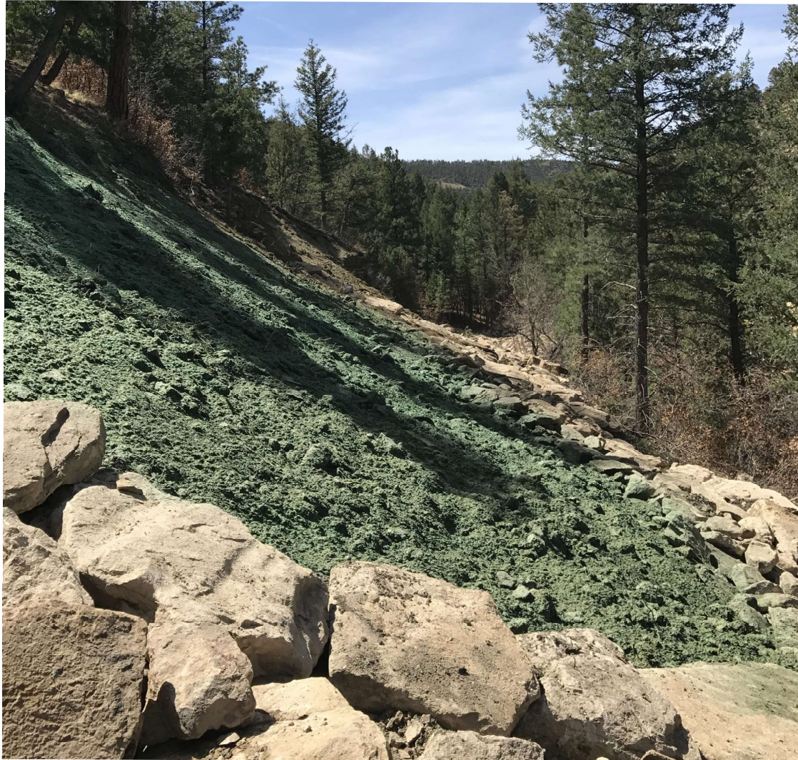
PHOTO 9: FACING SOUTHWEST TOWARD THE WELL PAD AND EAST PORTION OF THE GOLDEN EAGLE MINE E-1 AND E-2 ACCESS ROAD RECLAMATION. THE ACCESS ROAD WAS RECONTOURED TO MATCH THE SURROUNDING TERRAIN. GRADING TECHNIQUES WERE INSTALLED ON THE CONTOUR. ARMOR WAS INSTALLED TO RECEIVE RUN ON AND CONTROL EROSION. THE EARTH DISTURBANCE WAS HYDRO-SEEDED WITH AN APPROVED COLORADO PARKS AND WILDLIFE (CPW) SEED MIX TO PROMOTE THE ESTABLISHMENT OF VEGETATION.
