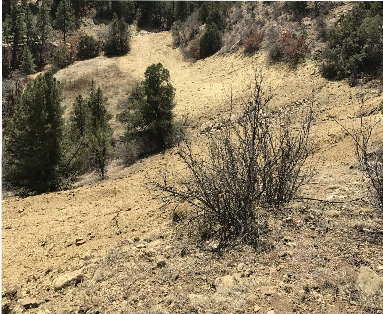
PHOTO 8: FACING SOUTH TOWARD THE WEST PORTION OF THE GOLDEN EAGLE MINE E-1 AND E-2 ACCESS ROAD RECLAMATION. THE ACCESS ROAD WAS RECONTOURED TO MATCH THE SURROUNDING TERRAIN. GRADING TECHNIQUES WERE INSTALLED ON THE CONTOUR. THE EARTH DISTURBANCE WAS HYDRO-SEEDED WITH AN APPROVED COLORADO PARKS AND WILDLIFE (CPW) SEED MIX TO PROMOTE THE ESTABLISHMENT OF VEGETATION.
