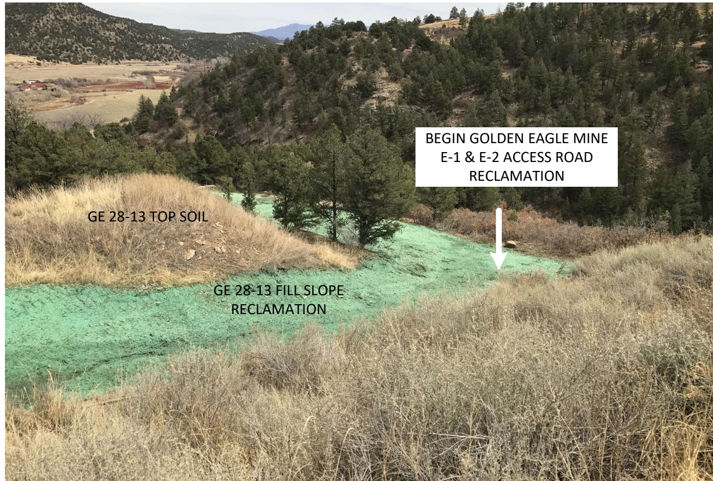
PHOTO 3 : FACING EAST TOWARD WELL PAD FILL SLOPE OF GOLDEN EAGLE 28-13 API # 071-06435. ACCESS TO THE WEST PORTION OF THE GOLDEN EAGLE MINE E-1 AND E-2 ACCESS ROAD RECLAMATION WAS GAINED FROM THE GOLDEN EAGLE 28-13 WELL PAD. THIS DISTURBANCE WAS RECONTOURED AND RECLAIMED. THE EARTH DISTURBANCE WAS HYDRO-SEEDED WITH AN APPROVED COLORADO PARKS AND WILDLIFE (CPW) SEED MIX TO PROMOTE THE ESTABLISHMENT OF VEGETATION.
