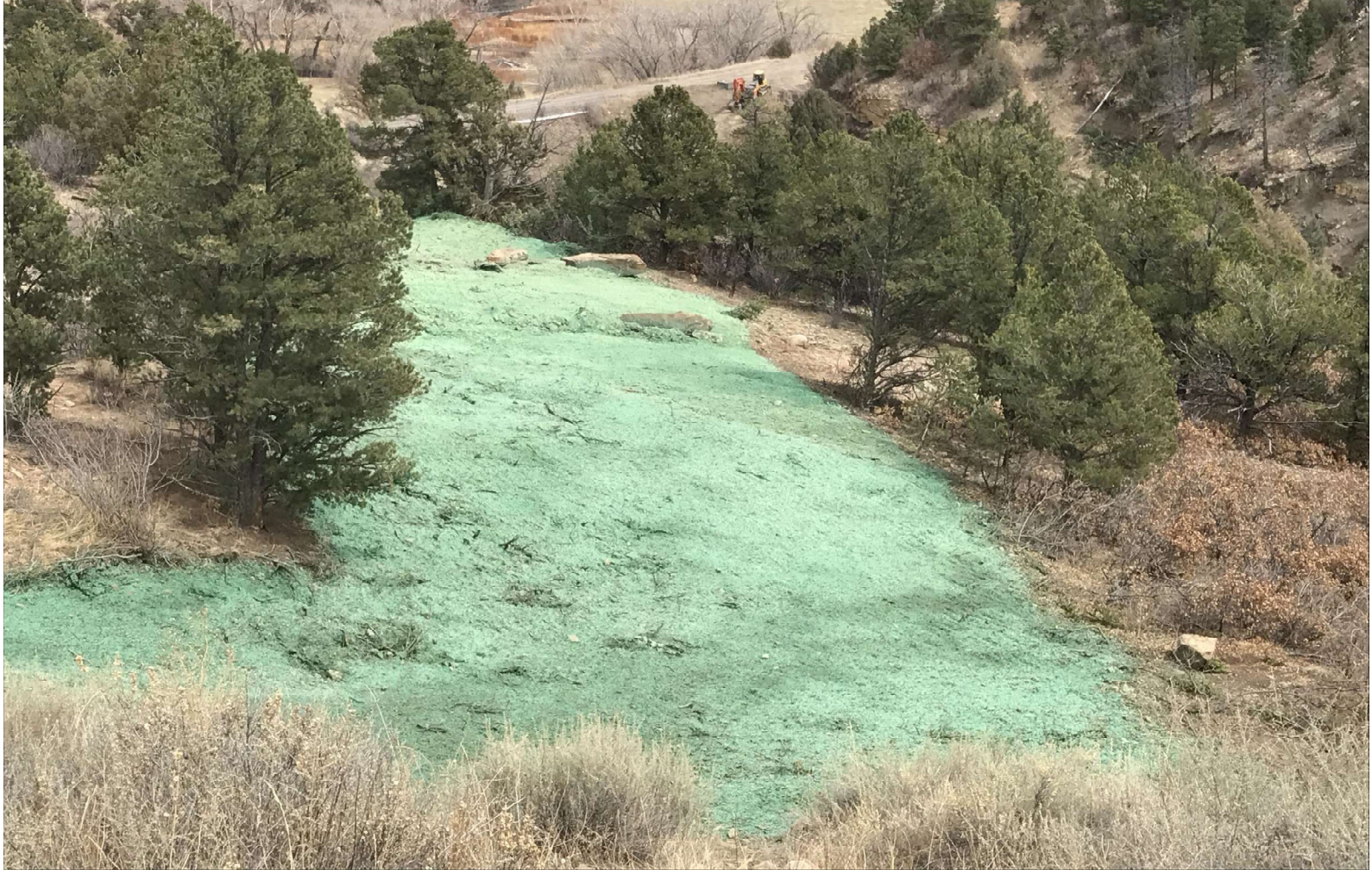
PHOTO 4 : FACING NORTHEAST TOWARD THE WEST PORTION OF THE GOLDEN EAGLE MINE E-1 AND E-2 ACCESS ROAD RECLAMATION. THE ACCESS ROAD WAS RECONTOURED TO MATCH THE SURROUNDING TERRAIN. GRADING TECHNIQUES WERE INSTALLED ON THE CONTOUR. THE EARTH DISTURBANCE WAS HYDRO-SEEDED WITH AN APPROVED COLORADO PARKS AND WILDLIFE (CPW) SEED MIX TO PROMOTE THE ESTABLISHMENT OF VEGETATION.
