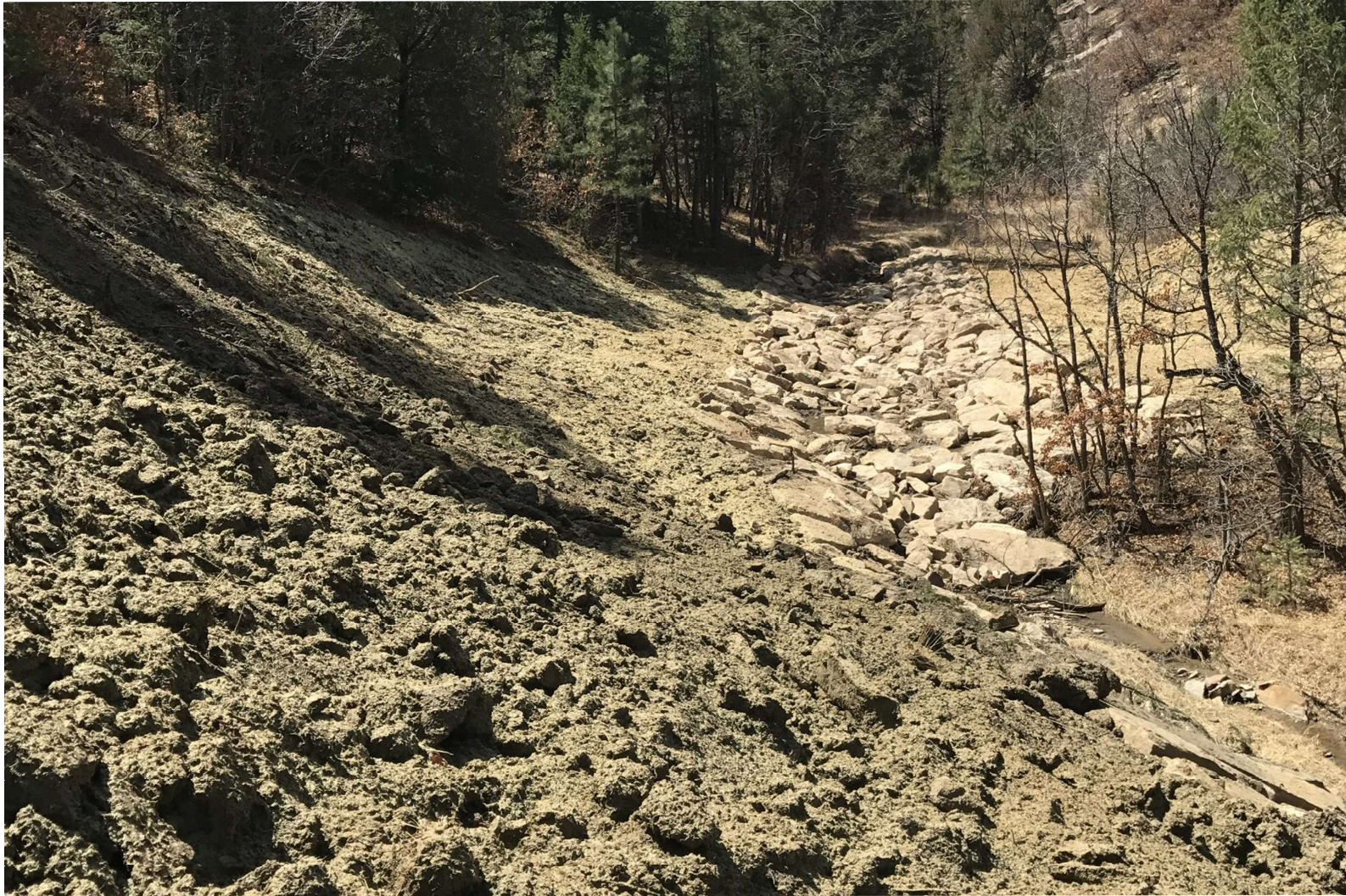
PHOTO 10: FACING THE CREEK BOTTOM OF THE GOLDEN EAGLE MINE E-1 AND E-2 ACCESS ROAD RECLAMATION. ALL PIPING, RISERS AND VALVES HAVE BEEN REMOVED. THE ACCESS ROAD WAS RECONTOURED TO MATCH THE SURROUNDING TERRAIN. GRADING TECHNIQUES WERE INSTALLED ON THE CONTOUR. ARMOR WAS INSTALLED IN THE CREEK BOTTOM FOR PERMANENT STABILIZATION. THE EARTH DISTURBANCE WAS HYDRO-SEEDED WITH AN APPROVED COLORADO PARKS AND WILDLIFE (CPW) SEED MIX TO PROMOTE THE ESTABLISHMENT OF VEGETATION.
