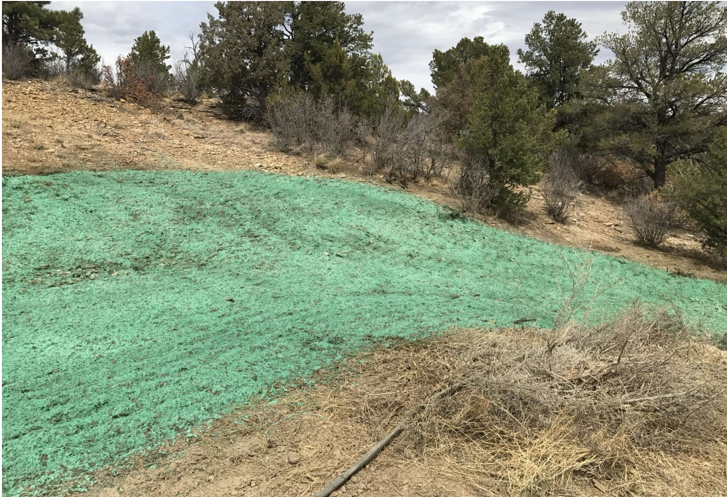
PHOTO 2 : FACING THE NORTH CUT SLOPE OF WELL PAD GOLDEN EAGLE 28-13 API # 071-06435 WERE THE CUT MEETS THE FILL SLOPE. ACCESS TO THE WEST PORTION OF THE GOLDEN EAGLE MINE E-1 AND E-2 ACCESS ROAD RECLAMATION WAS GAINED FROM THE GOLDEN EAGLE 28-13 WELL PAD. THIS DISTURBANCE WAS RECONTOURED AND RECLAIMED. THE EARTH DISTURBANCE WAS HYDRO-SEEDING WITH AN APPROVED COLORADO PARKS AND WILDLIFE (CPW) SEED MIX TO PROMOTE THE ESTABLISHMENT OF VEGETATION.
