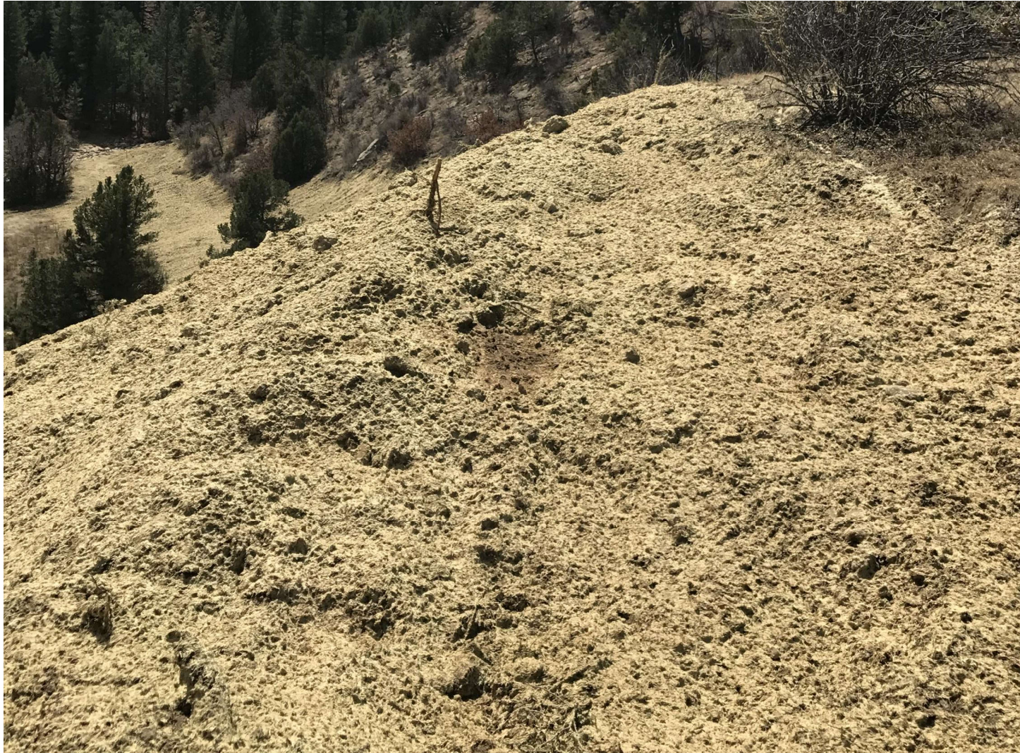
PHOTO 7: FACING SOUTH TOWARD THE WEST PORTION OF THE GOLDEN EAGLE MINE E-1 AND E-2 ACCESS ROAD RECLAMATION. THE ACCESS ROAD WAS RECONTOURED TO MATCH THE SURROUNDING TERRAIN. GRADING TECHNIQUES WERE INSTALLED ON THE CONTOUR. THE EARTH DISTURBANCE WAS HYDRO-SEEDING WITH AN APPROVED COLORADO PARKS AND WILDLIFE (CPW) SEED MIX TO PROMOTE THE ESTABLISHMENT OF VEGETATION.
