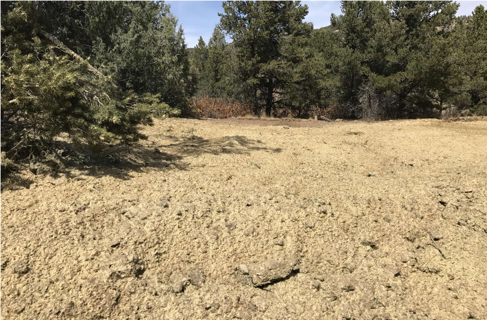
PHOTO 6 : FACING NORTH TOWARD THE WEST PORTION OF THE GOLDEN EAGLE MINE E-1 AND E-2 ACCESS ROAD RECLAMATION. THE ACCESS ROAD WAS RECONTOURED TO MATCH THE SOUROUNDING TERRAIN. GRADING TECHNIQUES WERE INSTALLED ON THE CONTOUR. THE EARTH DISTURBANCE WAS HYDRO-SEEDED WITH AN APPROVED COLORADO PARKS AND WILDLIFE (CPW) SEED MIX TO PROMOTE THE ESTABLISHMENT OF VEGETATION.
