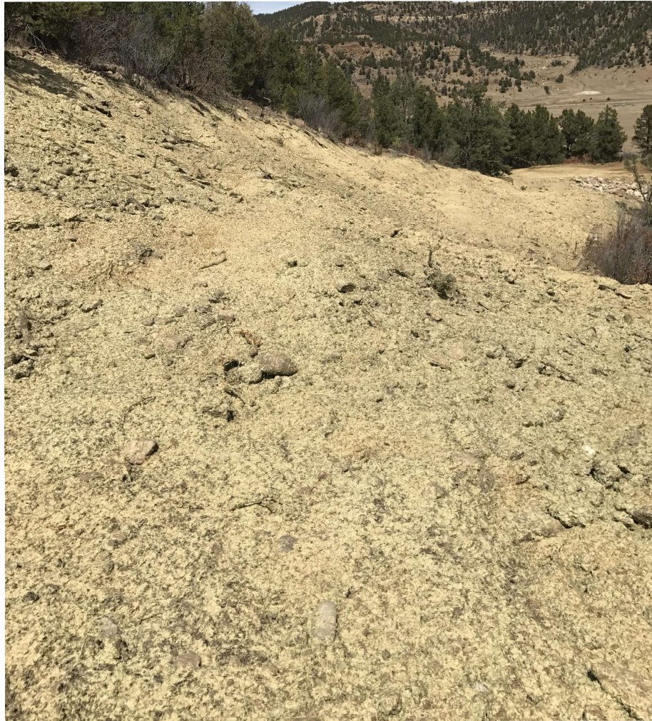
PHOTO 5 : FACING NORTH TOWARD THE WEST PORTION OF THE GOLDEN EAGLE MINE E-1 AND E-2 ACCESS ROAD RECLAMATION. THE ACCESS ROAD WAS RECONTOURED TO MATCH THE SURROUNDING TERRAIN. GRADING TECHNIQUES WERE INSTALLED ON THE CONTOUR. THE EARTH DISTURBANCE WAS HYDRO-SEEDED WITH AN APPROVED COLORADO PARKS AND WILDLIFE (CPW) SEED MIX TO PROMOTE THE ESTABLISHMENT OF VEGETATION.
