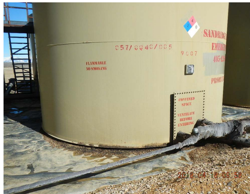
Oil staining on gravel near Tank # 9007
