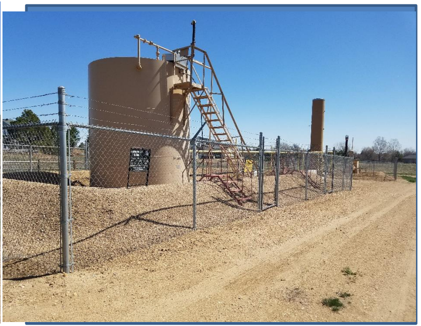
Photo 2. Tank battery
