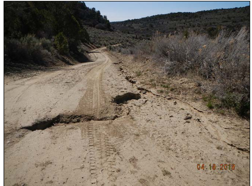
Photo 4. Erosion of access road and sediment migration down gradient.
