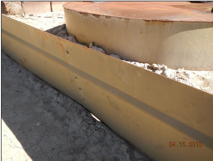
Photo 3. Tank containment is inadequate.
