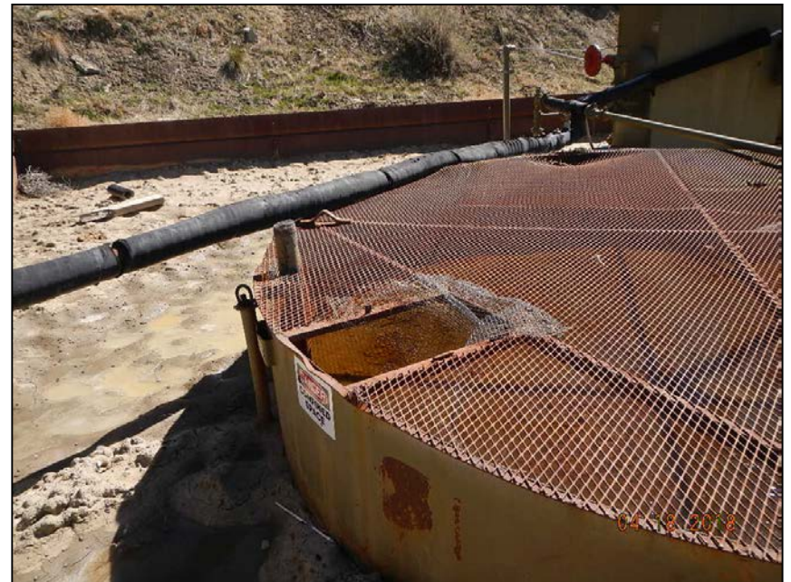
Photo 2. No sign on open tope tank. Bird protection is damaged.
