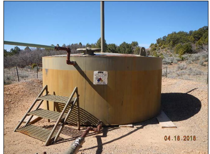
Photo 2. Produced water tank.
