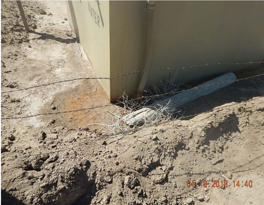
Photo 9: Stained soil around water vault.
