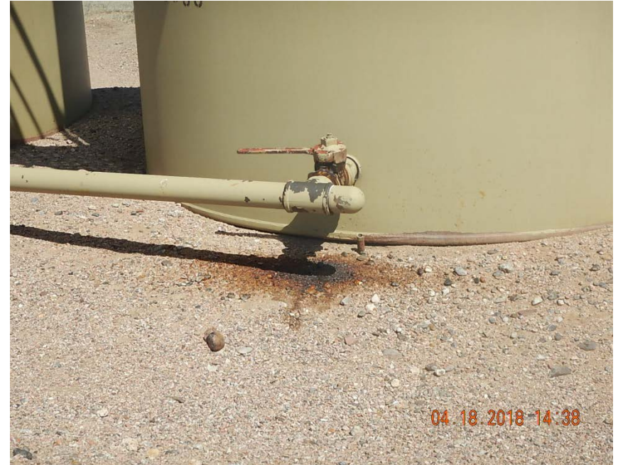
Photo 6: Stained soil at loadout.
