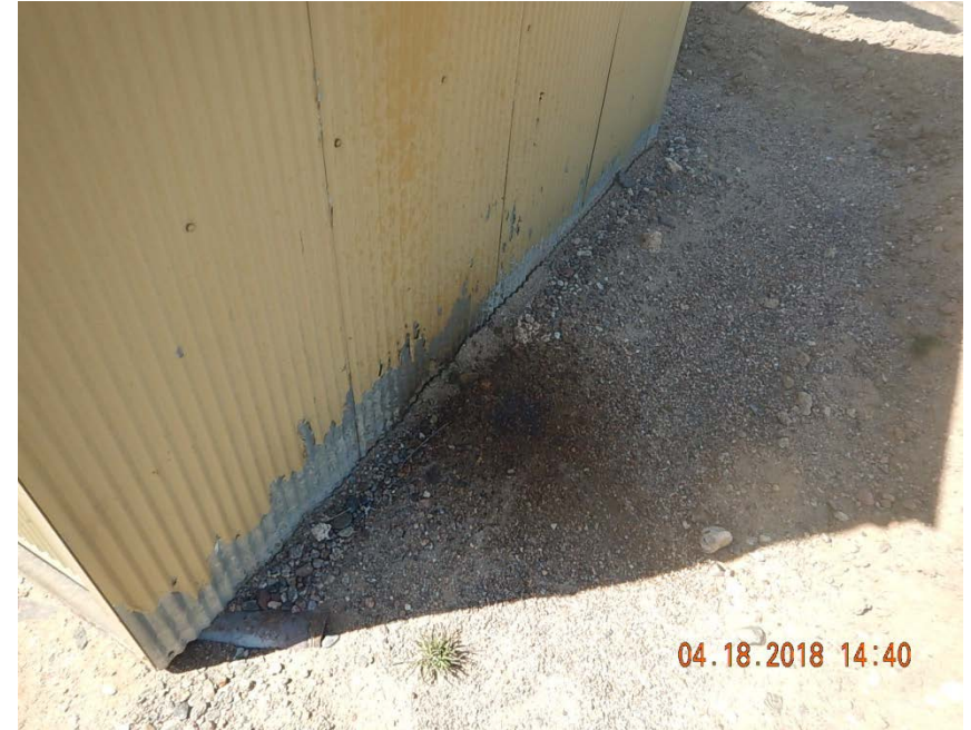
Photo 8: Stained soil on E side of treater house
