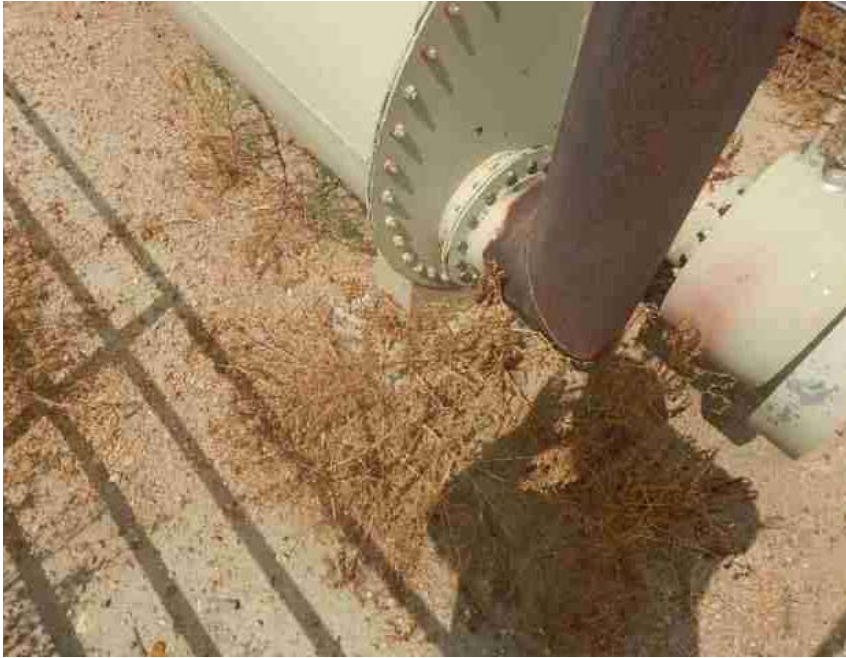
Photo from prior inspection for comparison
