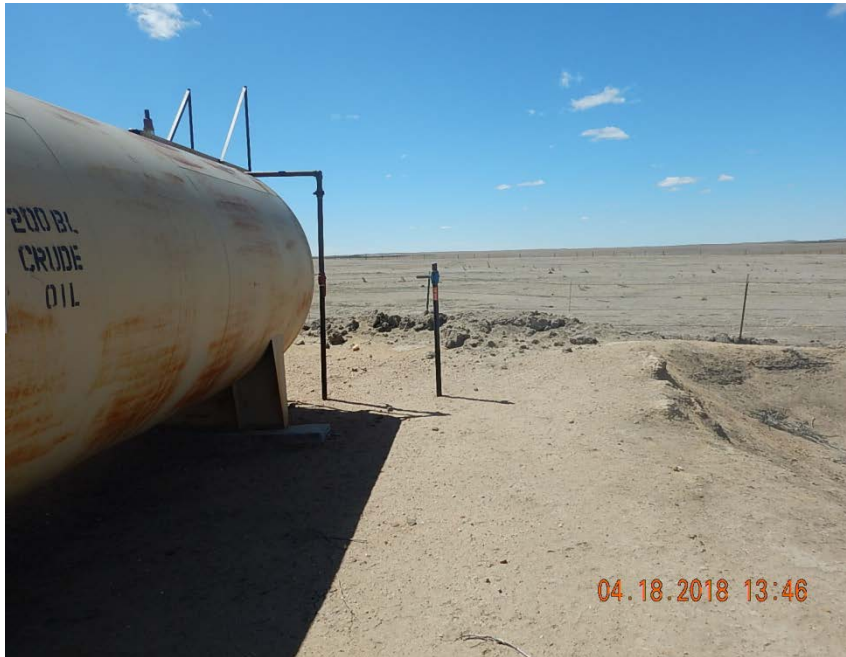
Photo 8: In use, plugged flowline riser.
