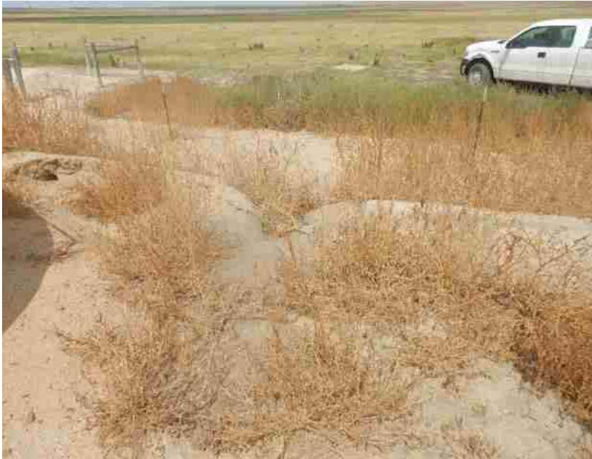
Photo from prior inspection for comparison
