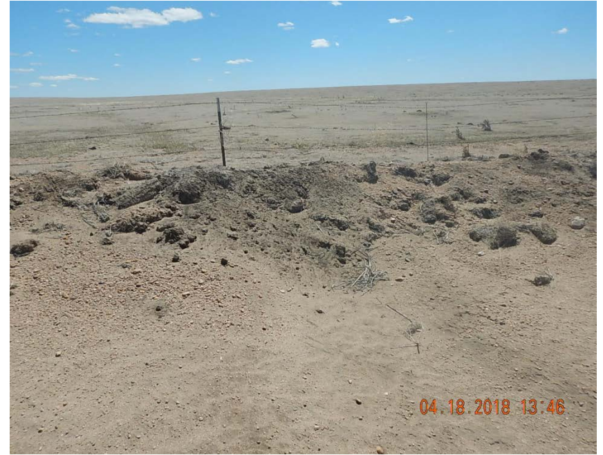
Photo 7: Stormwater erosion mitigated.
