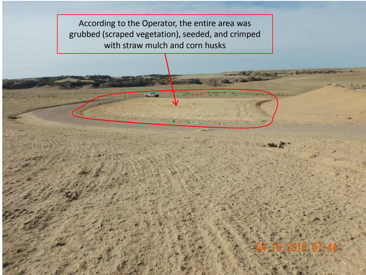
Photo 12. Photo taken east of the well pad perimeter, facing South. Photo illustrates impacts of wind erosion sediment deposition. Existing and seeded vegetation in the photo foreground was not apparent and is covered with soil particles from wind erosion sediment deposition. This is also apparent for the red highlighted area.
