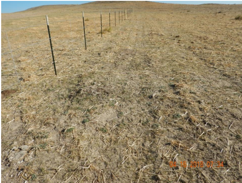
Photo 8. Photo taken from the southeast fence corner, facing North. See comments under Photo 6. Straw mulch did not appear to stay crimped throughout the location and has moved from the target areas, and will not function properly.
