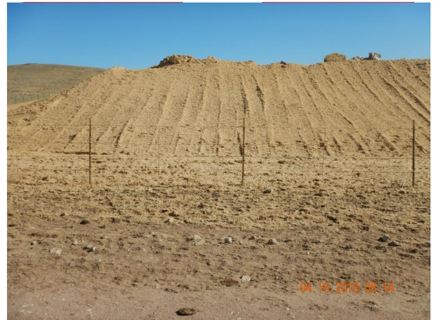
Photo 4. Photo taken from the southwest perimeter of the location, facing North. Photo illustrates fill slopes where there does not appear to be impacts from wind erosion sediment deposition.
