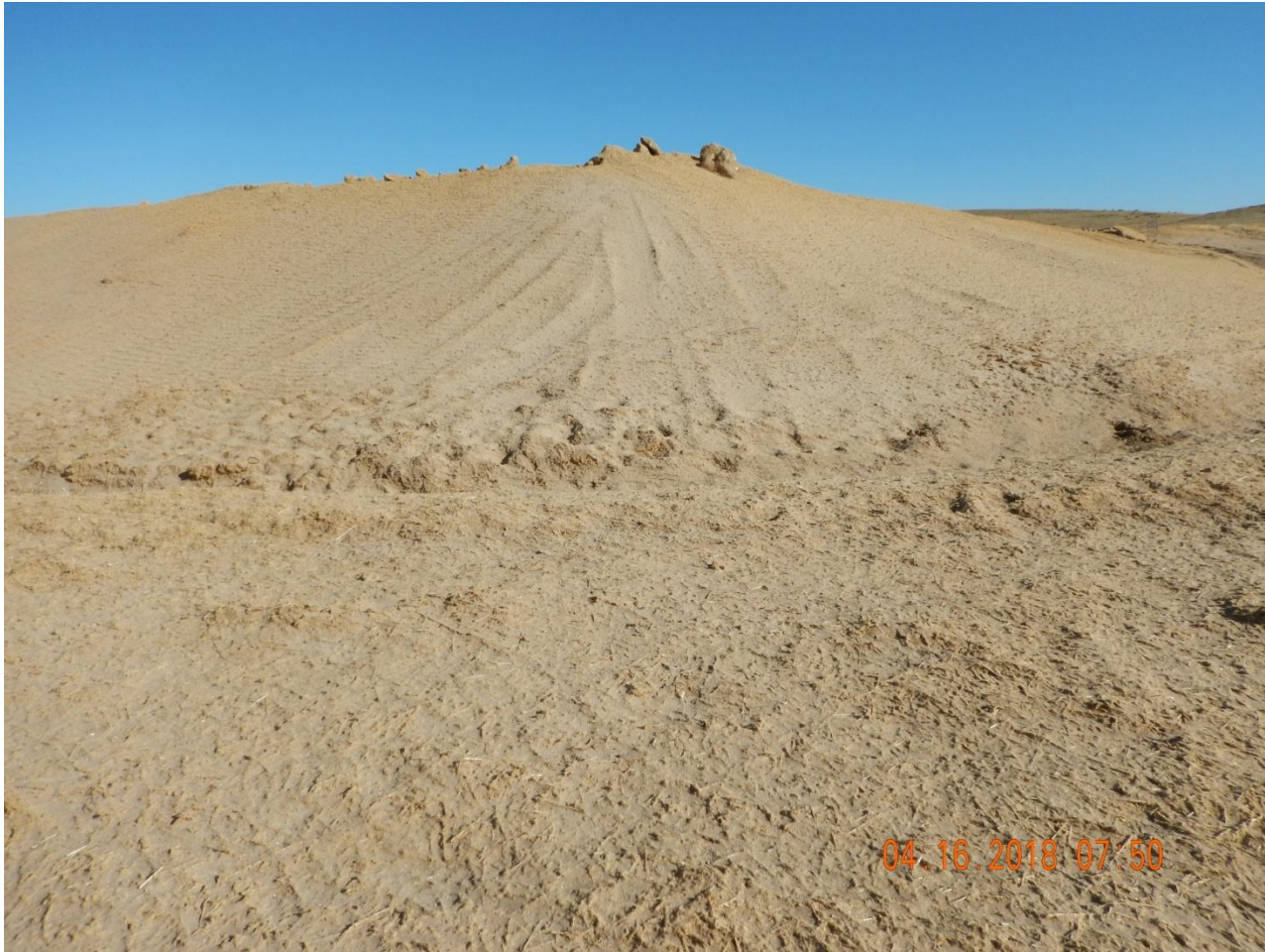
Photo 2. Close-up photo taken of the southeast fill slope area, facing Northwest. Photo illustrates evidence of wind erosion sediment deposition on fill slopes from unconsolidated well pad areas.
