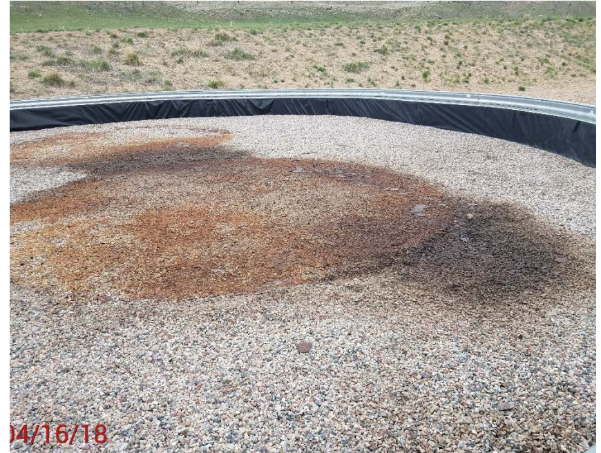
Location Photo # 6, Stained material in containment.
