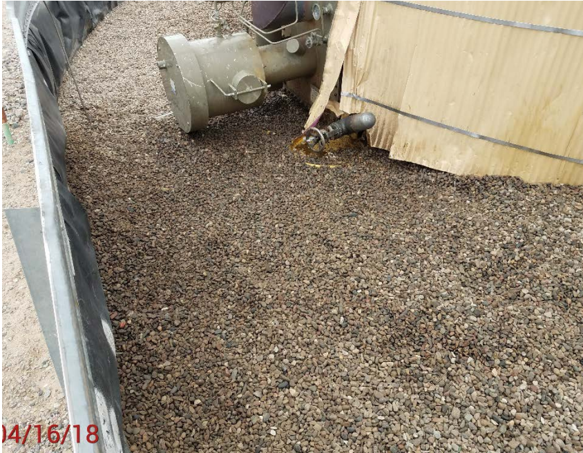
Location photo # 5, Standing Condensate in drip pan near a fire source.
