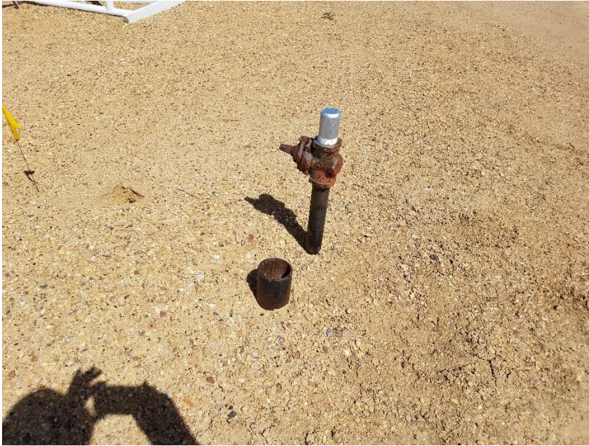
Photo 5. Unmarked riser at meter house
