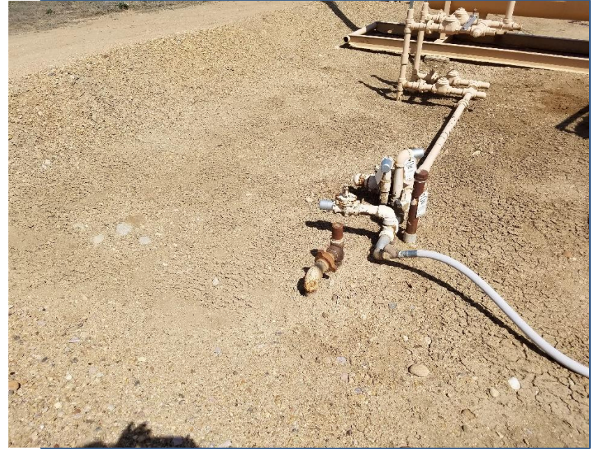
Photo 6. Unmarked riser near separator
