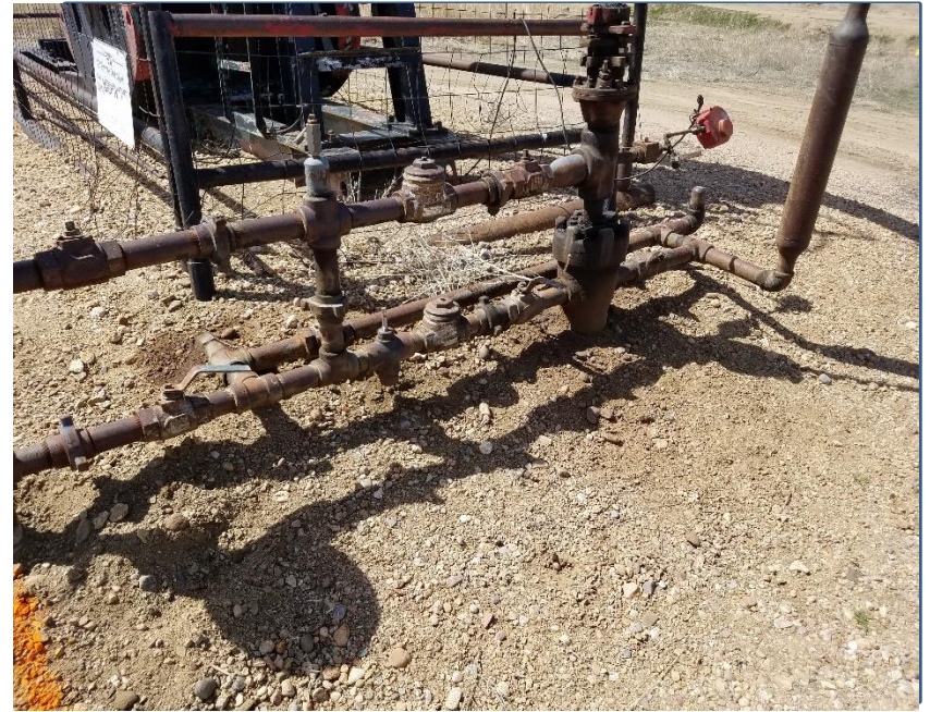
Photo 8. Stained soil around C. #1 wellhead
