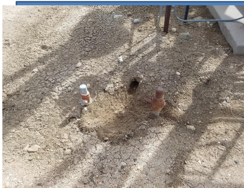
Photo 2. Unmarked risers
