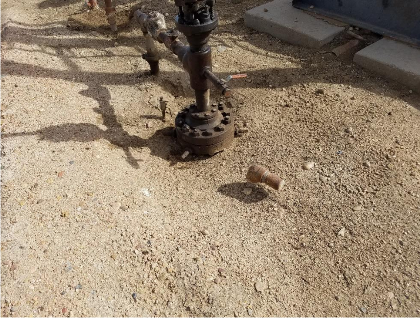
Photo 3. Unmarked riser
