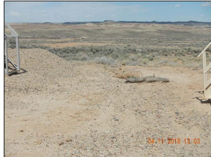
**Photo 2. Sediment leaving location through wattle that has become debris.**
