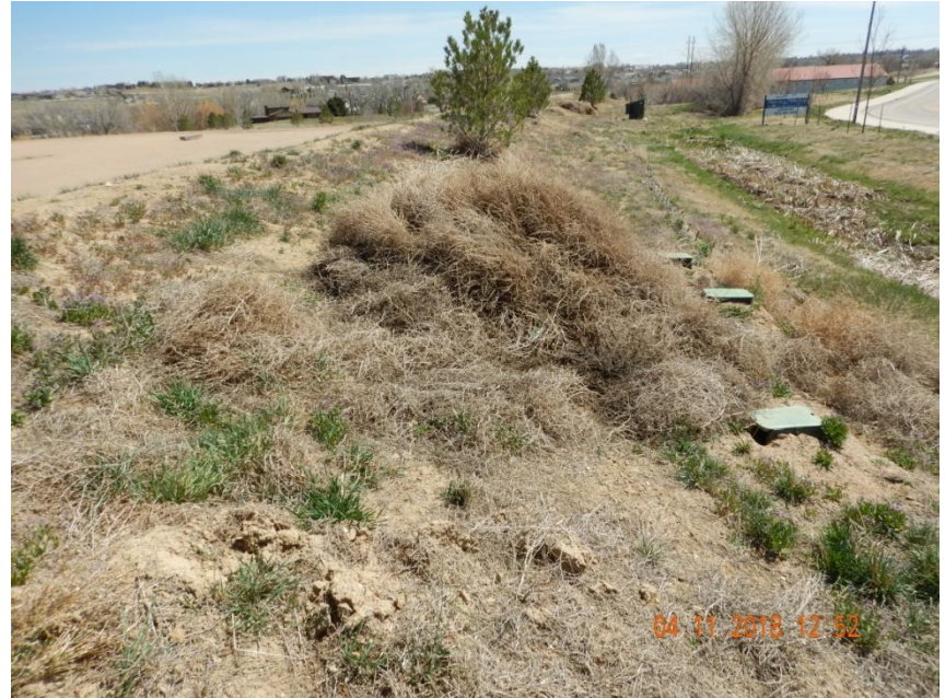
Photo 2. Photo taken from the southwest location, facing East. See comments under Photo 1. In addition, there does not appear to be sufficient perennial vegetation along the south-facing slope along the southern location.
