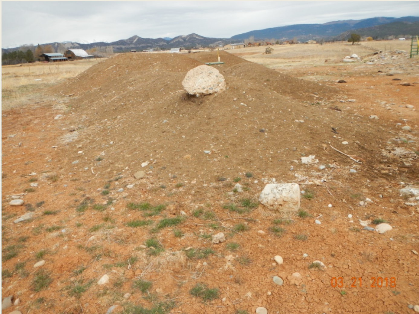
Photo 5. View of soil piles in the western project area. Cement debris, metal, and liner debris observed within the piles.
